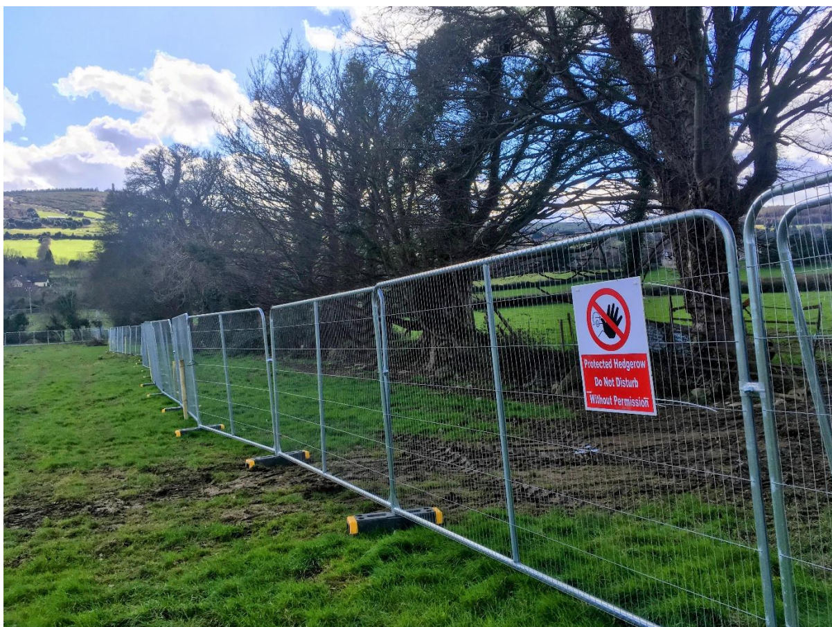
Figure 6 Fencing erected to prevent machinery working close to hedgerows
