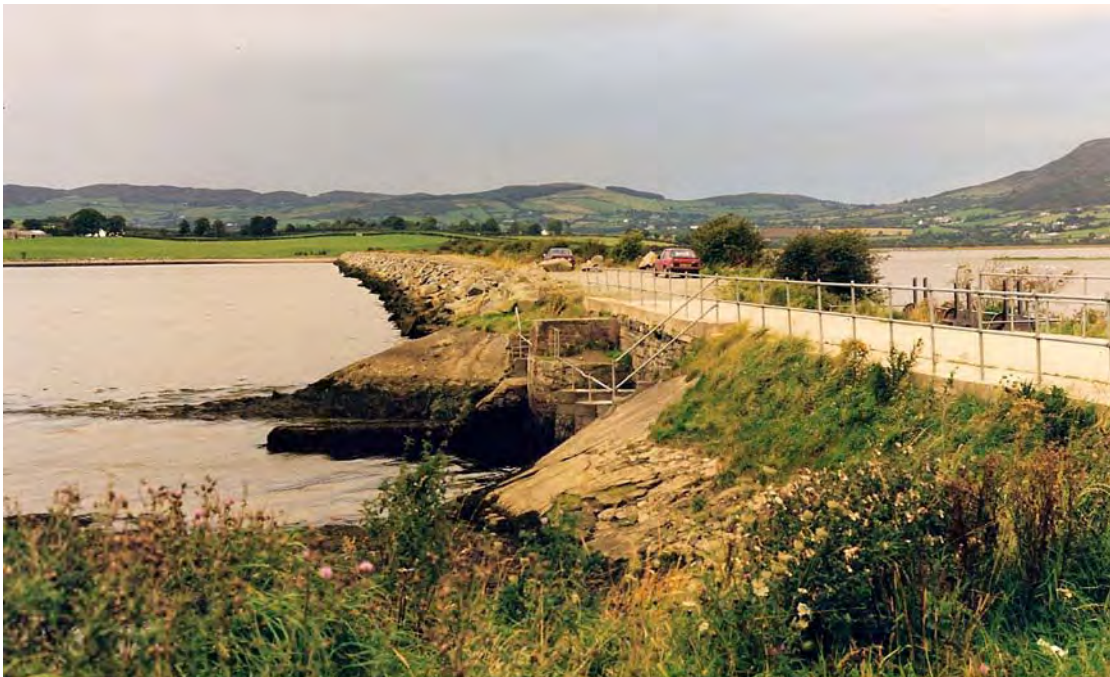
Plate 10. Inch Lough, County Donegal, an artificial lagoon. Showing the barrier and non-return valves.
