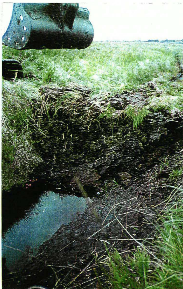
Plate 11. Half of the dam built from one side of a wide channel in Ballangare Bog.
