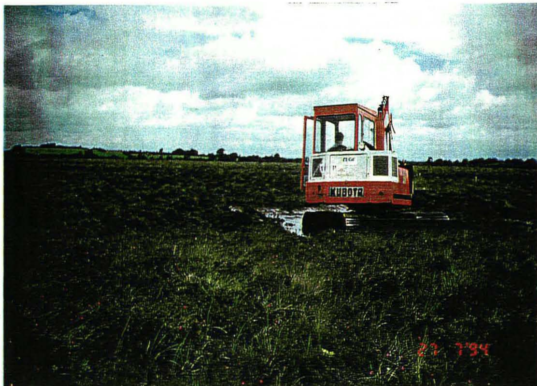
Plate 5. Machine working on mats on Garriskil Bog. July 96'
