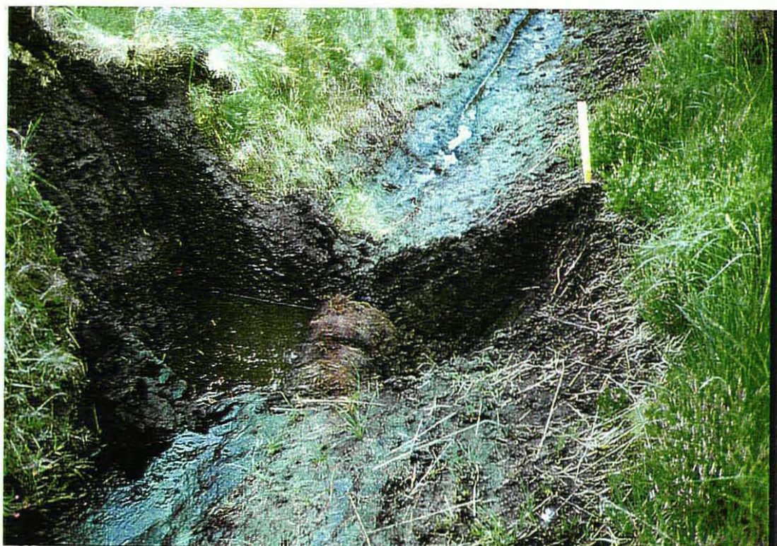
Plate 10. Placing of peat in the drain.
