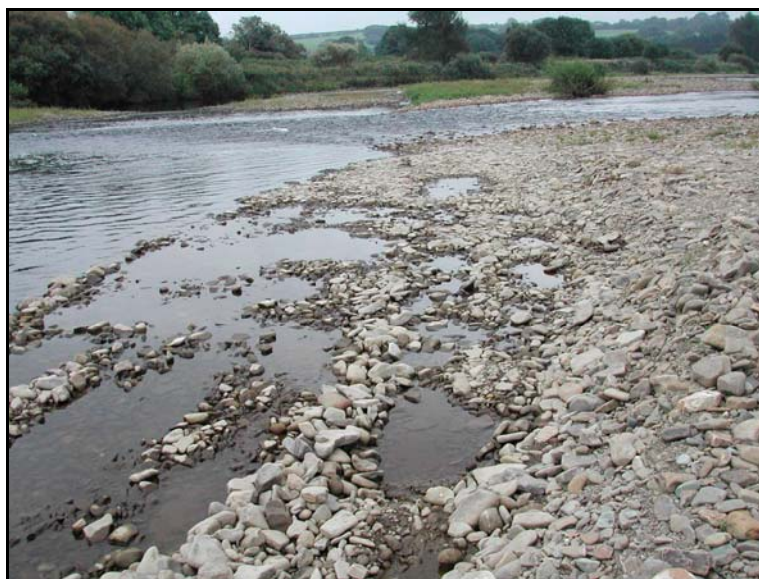
Plate 4 Evidence of recent gravel removal on the main River Feale upstream of Duagh Bridge.
