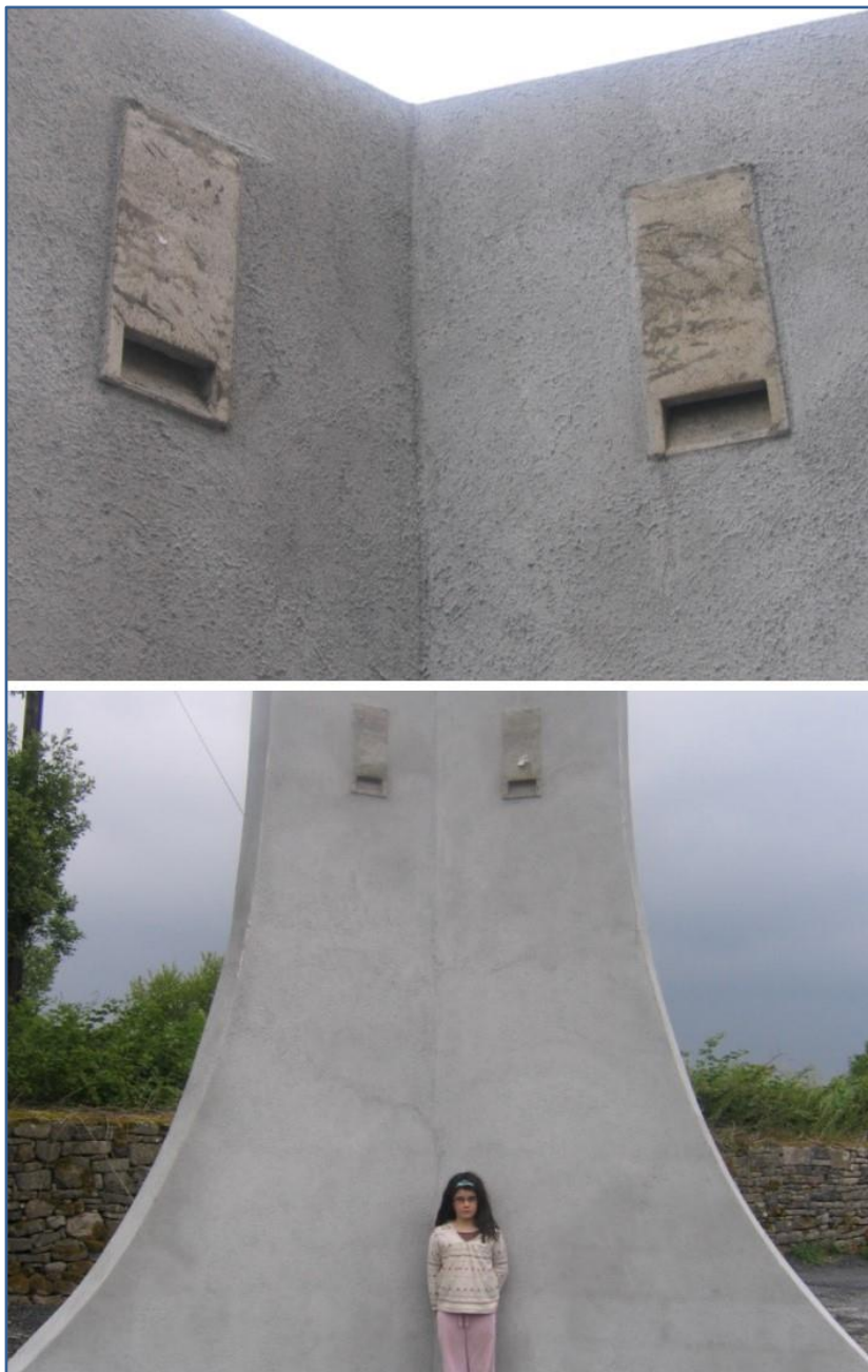
Figure 26 This structure was built at Errit Lake, Co. Roscommon to compensate for an old house which was demolished in 2010. There are six Schwegler bat tubes built into the structure. A small number of Daubenton's bats had been recorded roosting in the house. Last time it was checked the bat tubes were being used by Soprano pipistrelles. [Photographs: Caroline Sheils]
