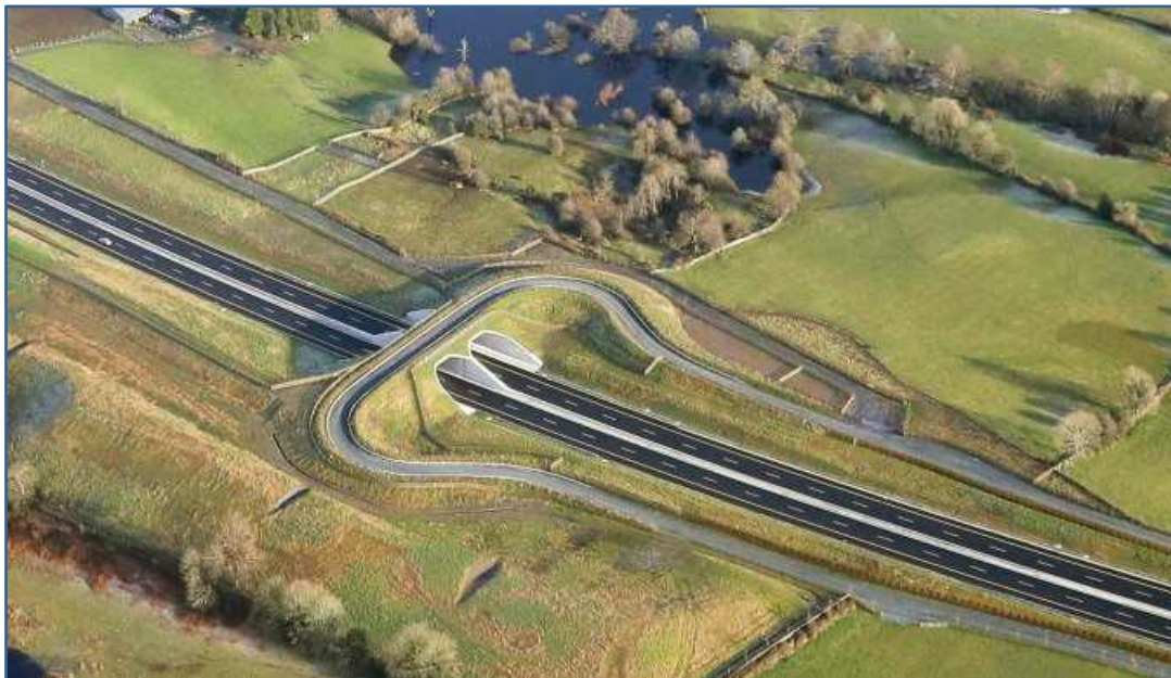
Figure 29 Ireland’s first green bridge built over the M17/18 to mitigate against the barrier caused by the road to lesser horseshoe bats commuting to their feeding grounds. It is a dual purpose green bridge and farm overpass. (Acknowledgements Galway Co. Co and Tina Aughney)
