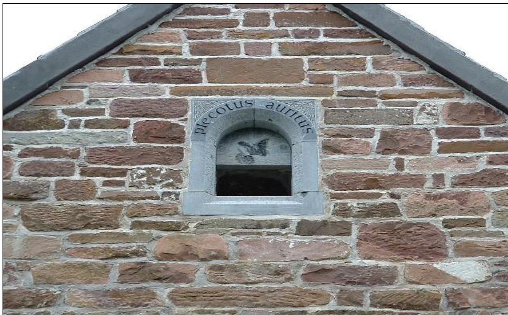
Figure 25. Roost entrance for brown long-eared bats but also large enough for lesser horseshoe bats. [Photograph: Conor Kelleher]
