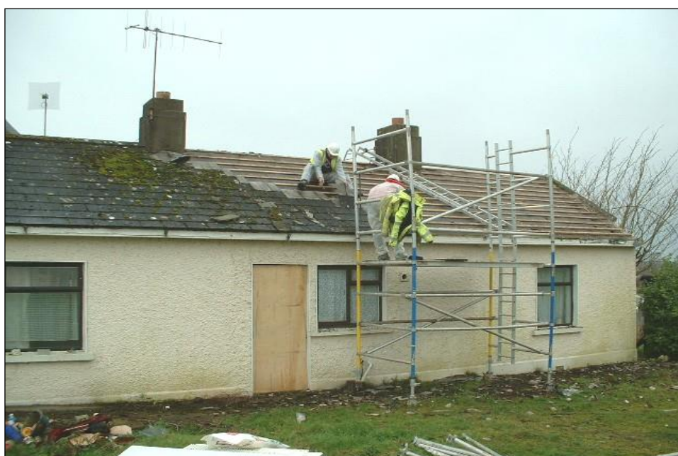
Figure 24 Re-roofing operations may require timing restrictions. [Photograph: Conor Kelleher]
