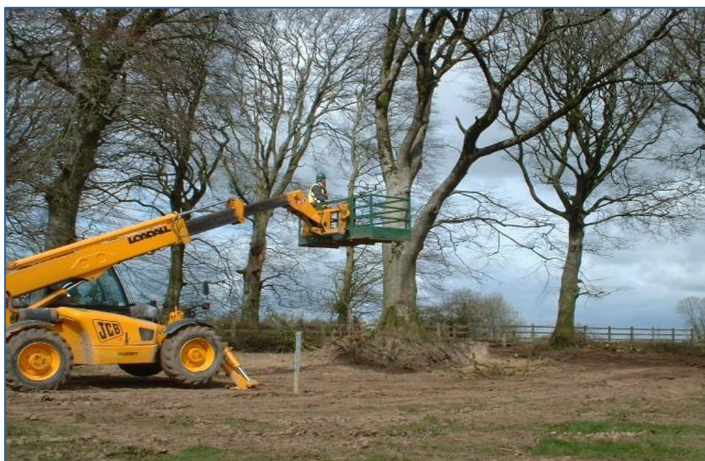
Figure 1 Tree removal by manual dismantling to safeguard bats. [Photograph: Conor Kelleher]
