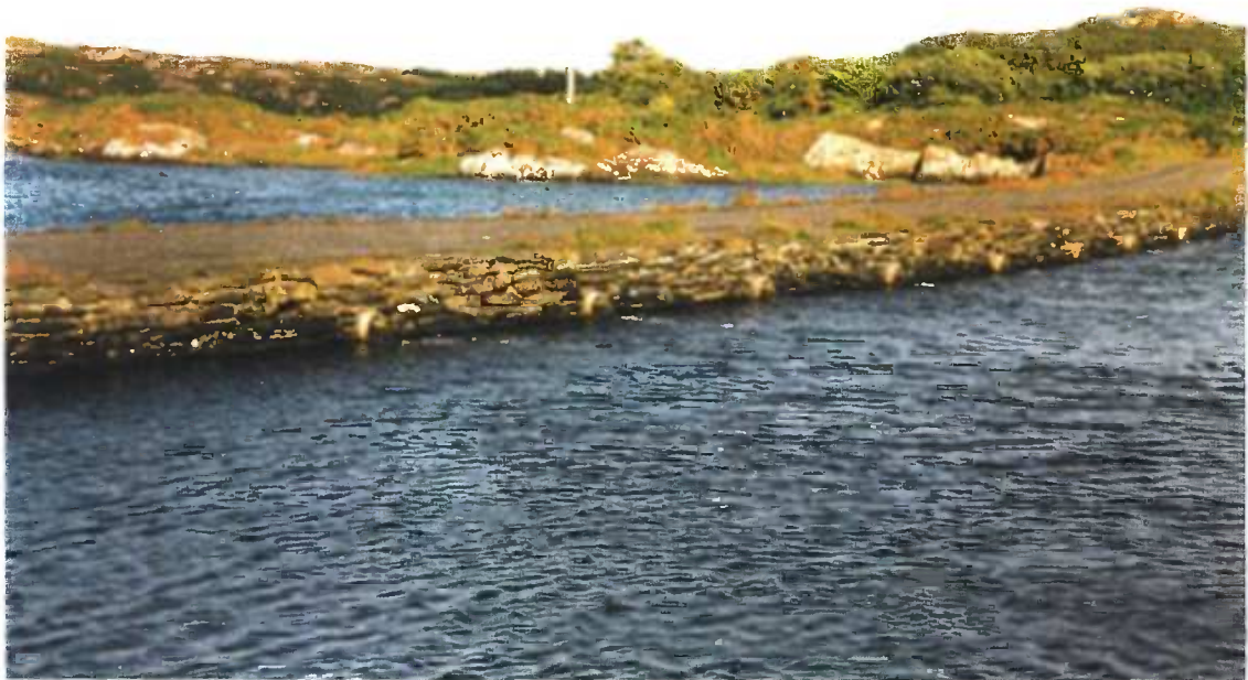
Toormore Lake. Causeway with outlet pipes
