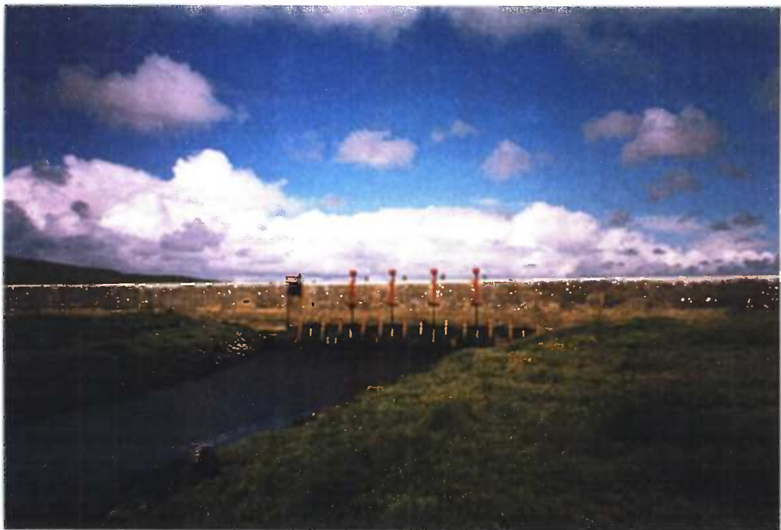
Lough Akeragh. Artificial barrier and sluice gates.
