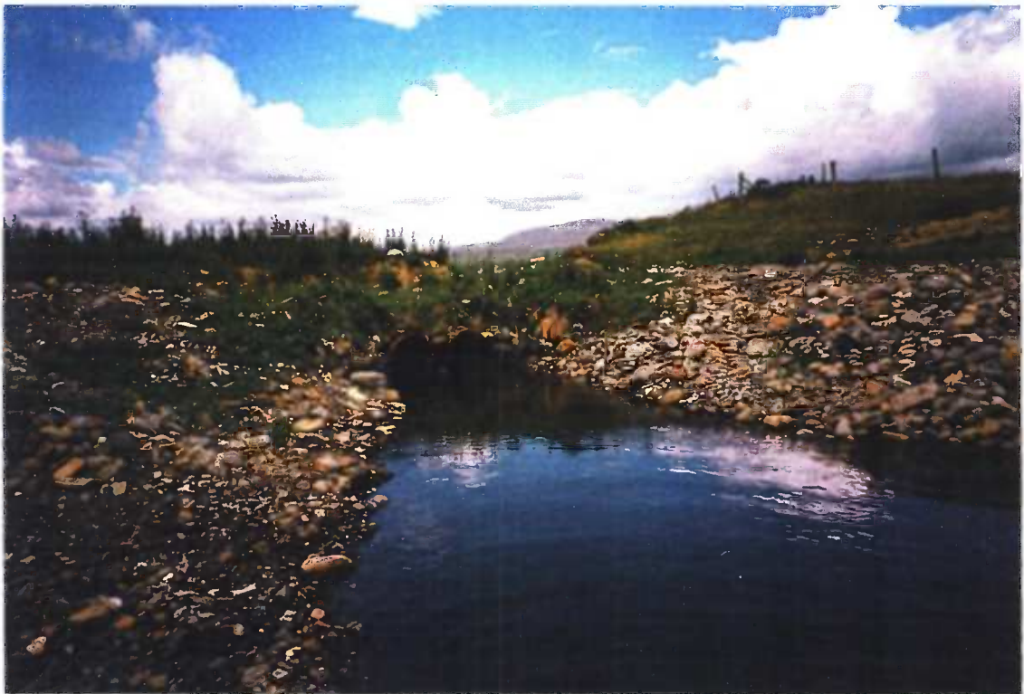
Reenydonagan Lake. Outlet pipes through the barrier.
