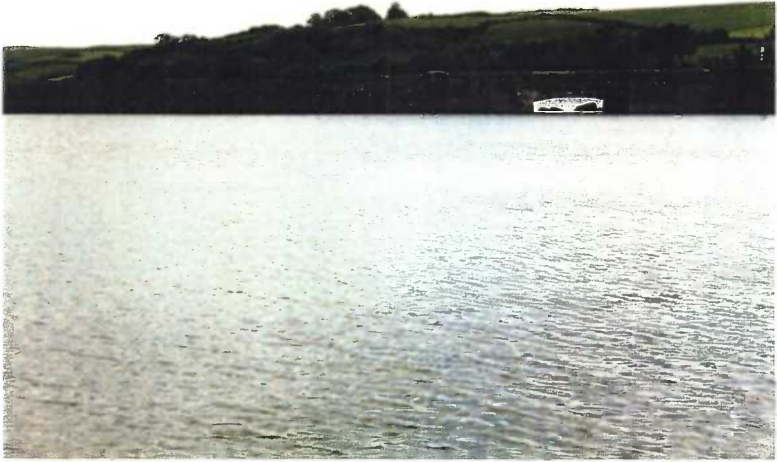
Rosscarbery Lake. Causeway and bridge over inlet.
