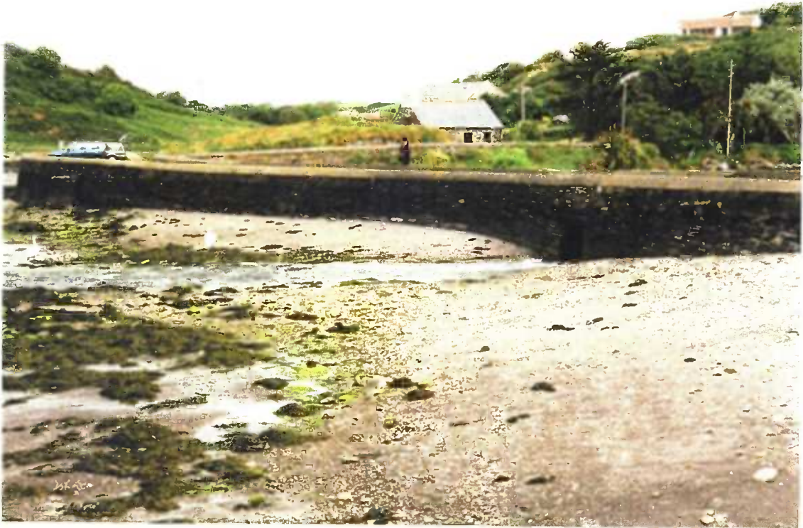
Blind Harbour. View of causeway and outlet to the sea.
