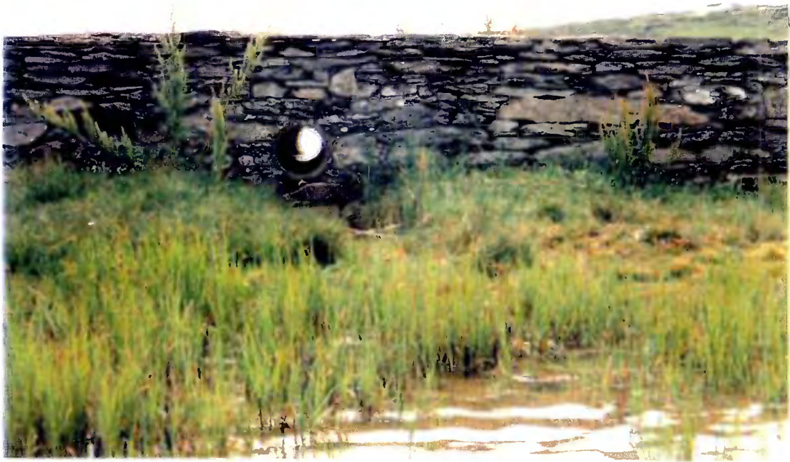
Plate 4.2.3 View of one of the pipes leading through the causeway of Lissagriffin Lake, Station B
