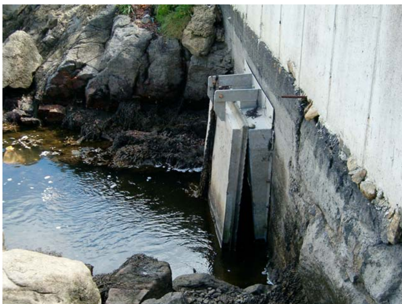
New steel sluice gate installed at Maghery Lough in 2003 by Donegal County Council (photo Emer Magee).
