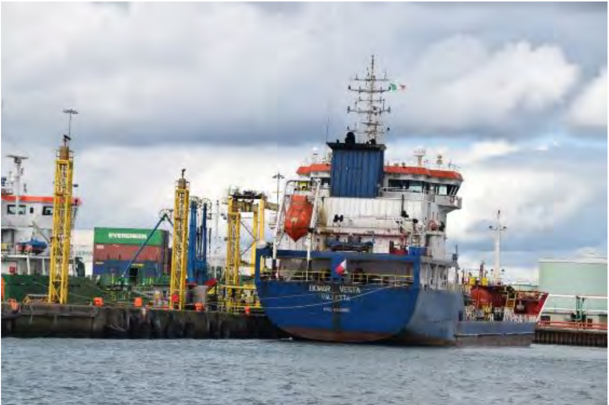
Plate 3-4 Western Oil Jetty - Oil Berth 2
