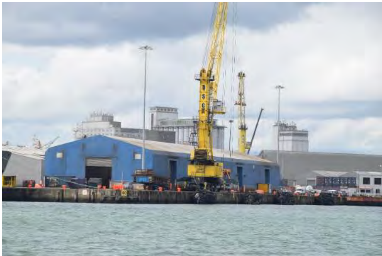
Plate 3-3 Berth 36 and Berth 37 (Ocean Pier), Alexandra Basin East
