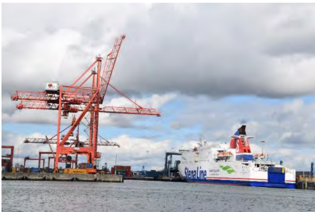
Plate 3-6 Ferryport Basin used for Ro-Ro freight & passenger and Lo-Lo freight operations
