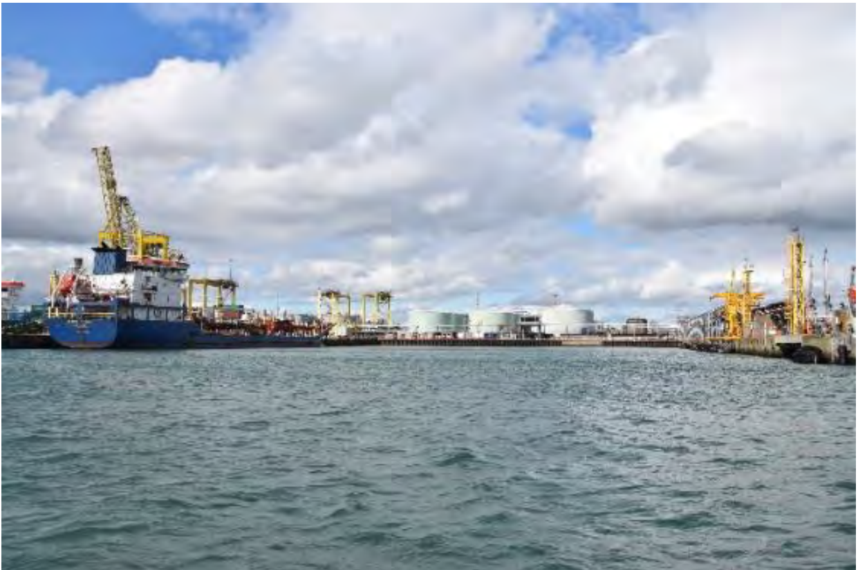
Plate 3-5 Oil Basin between Oil Berth 2 (left) and Oil Berth 3 (right)
