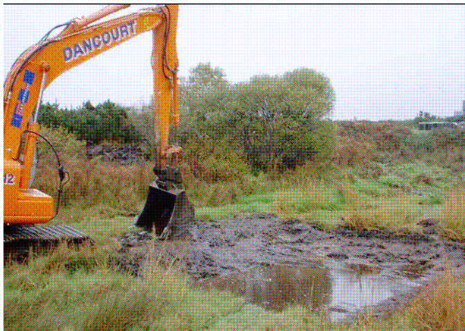
A new pond being dug for toads near Castlemaine
