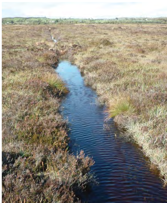
Plate 4.2 After peat dams drain blocking at Cuckoo Hill raised bog (Co. Roscommon) by Bord na Móna
