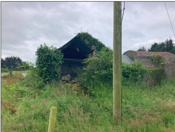
Plate 2 Rear of Shed 2 - bat droppings were found on an interior wall - note Japanese knotweed in front of shed.
