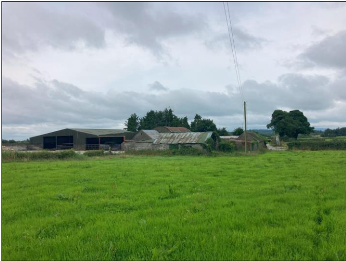
Plate 1 View of site from NE - note modern cow shed on the left. Shed 2 is in the foreground. The mature trees in the background don't present a lot of potential for bat roosts.
