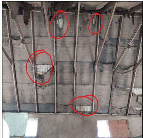
Plate 26: Gaps between gaps between a felt underlay and the asbestos roof in S10
