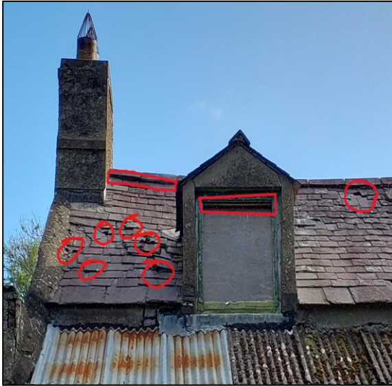
Plate 15: PRFs in a gap between window frames in a tow-storey structure in S06
