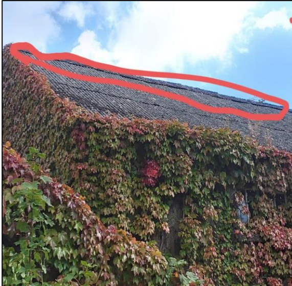
Plate 39: Gaps between ridge and roof panels provide PRFs in S14
