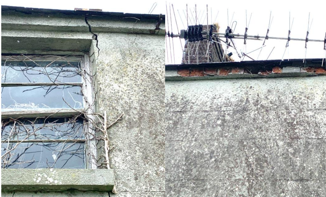
Figure 4. Cracks in masonry and render creating cavities and potential access points to interior of house.
