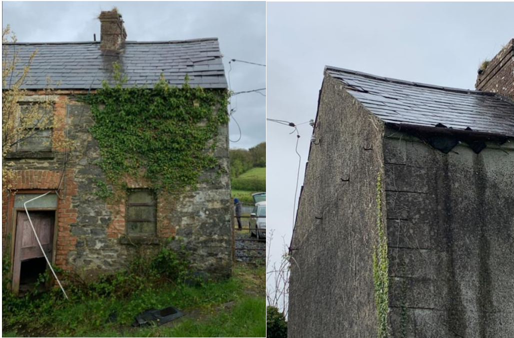
Figure 3. Loose slates on the N and S side of the roof.
