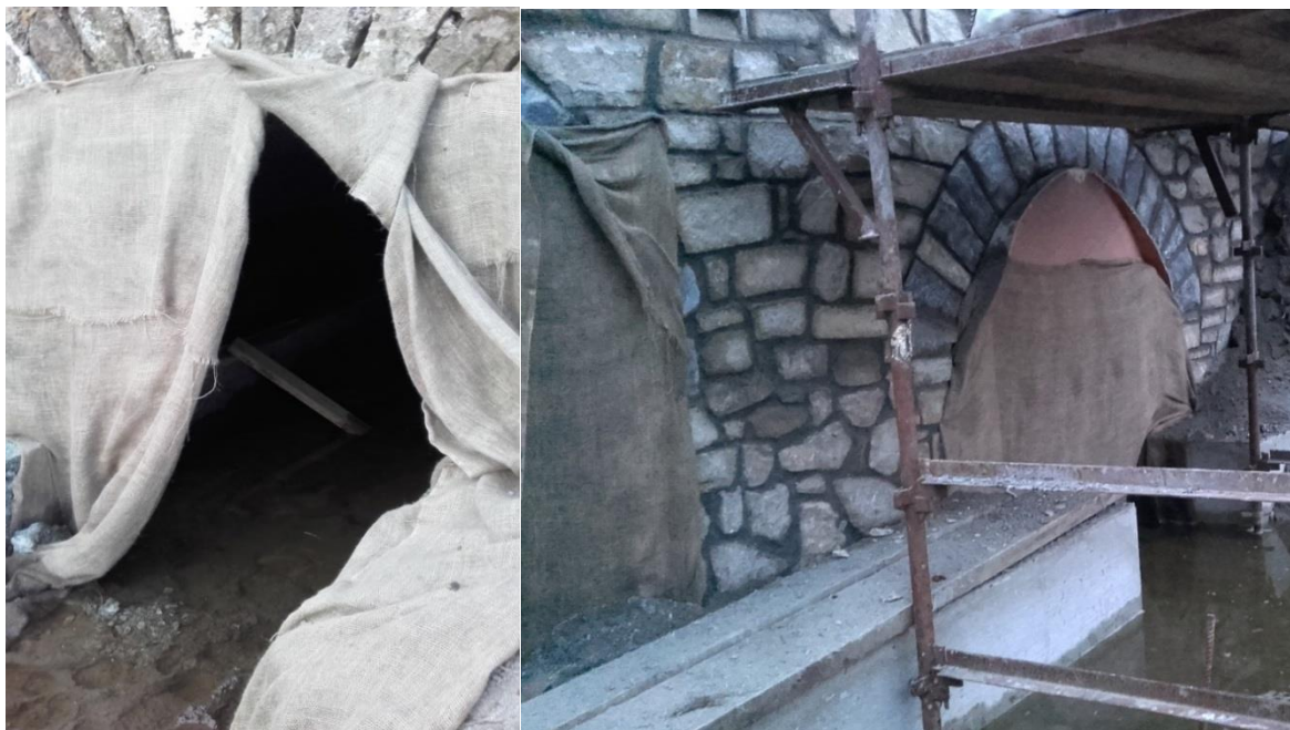
Plates 6a, b Example of hessian material curtains for sealing bridge arches
