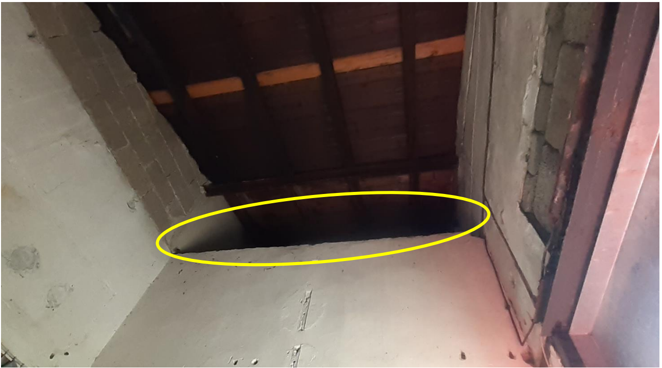
Plate 6: Internal wall in between the two rooms (Part C and Part D) of Substation Room. (Yellow Circle).
