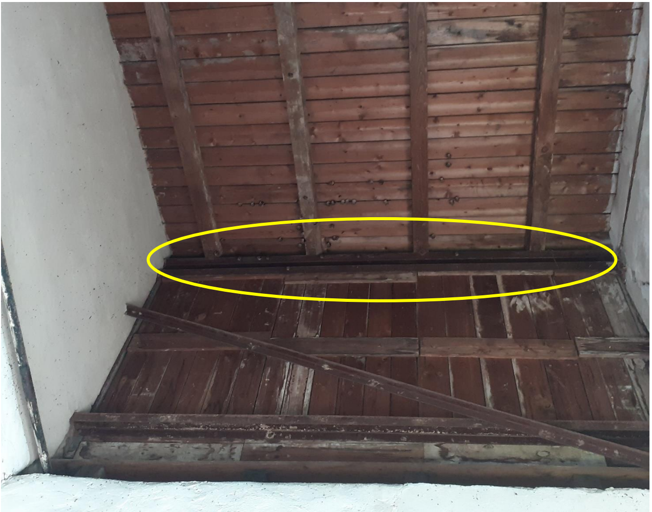
Plate 3: Rafter space in Part C, Substation Room (Lesser horseshoe bats visible – highlighted in yellow).
