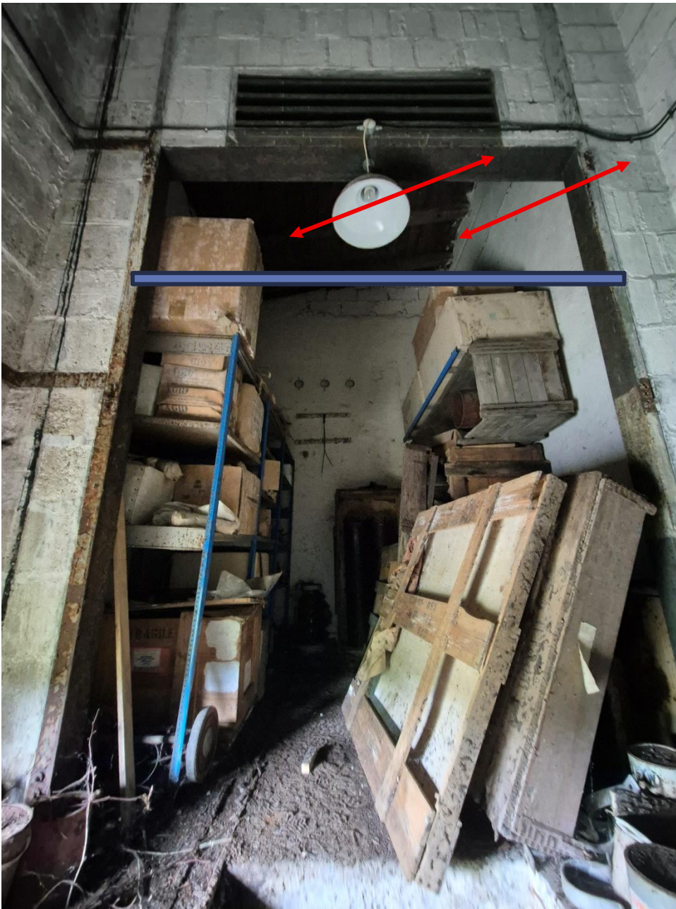
Plate 18: Room B of Transition Room.
