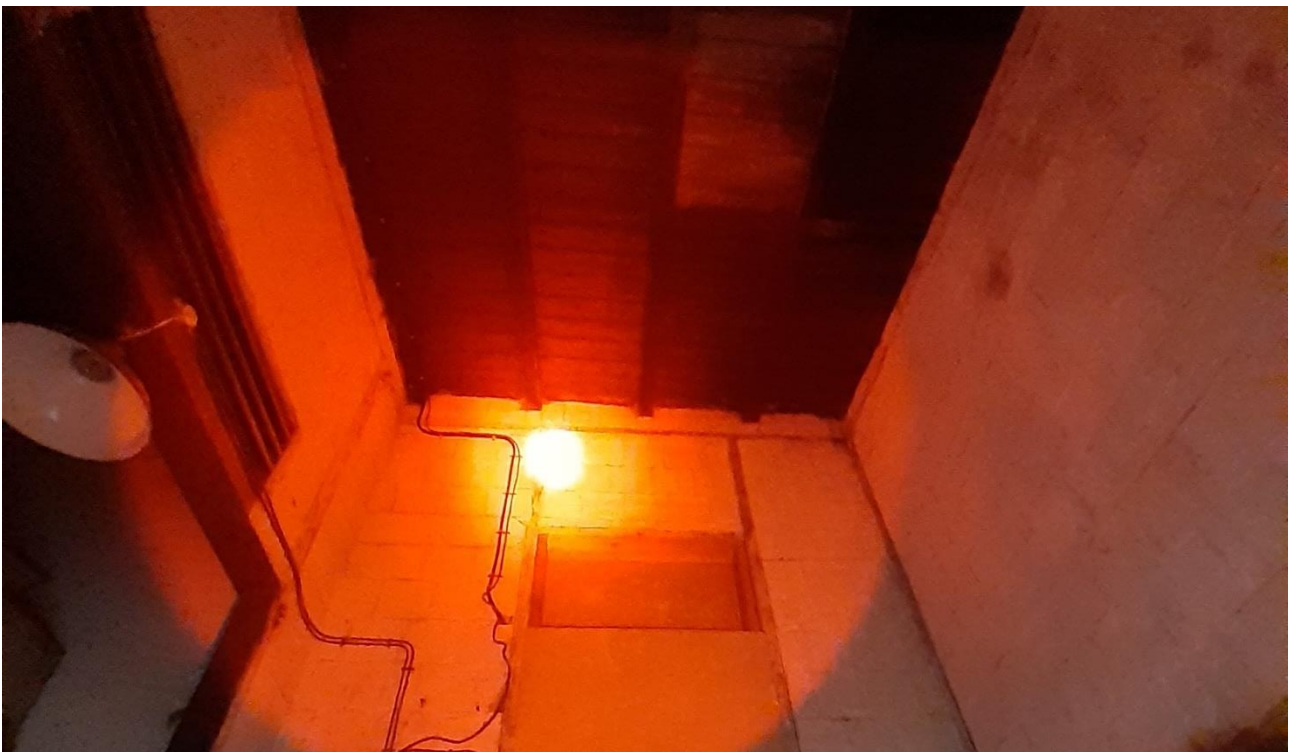
Plate 9: Internal space of Part A, Transition Room (depicting the wall shared with the main space of the Transformer Building. Entrance/Exit into the main space of the Transformer Building is at the rafter level highlighted by the Red Torch.
