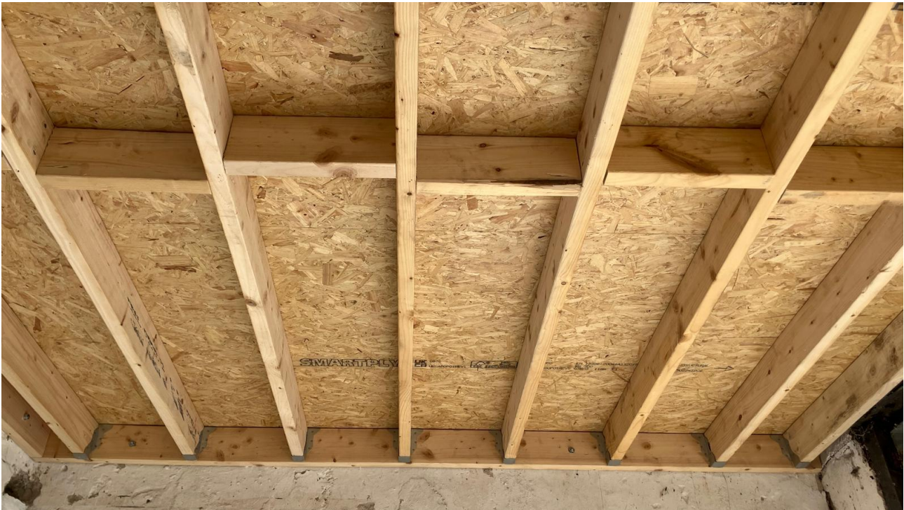
Plate 12: The underside of new loft floor completed on 30 th April 2025.
