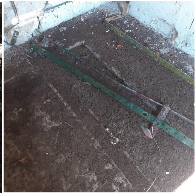
Plate 5: Extent of old bat droppings present on the substation floor (Part C).
