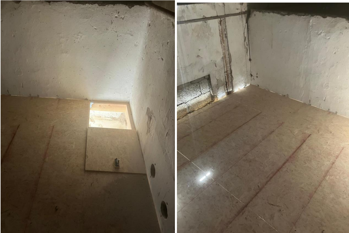
Plate 11a,b: New loft floors completed on 30 th April 2025.
