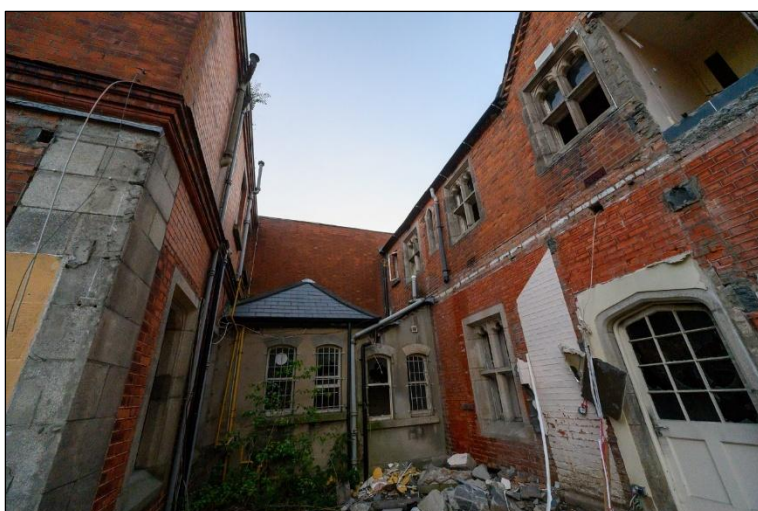
Plate 8 Courtyard at the rear of St. Joseph's house, June 2025.
