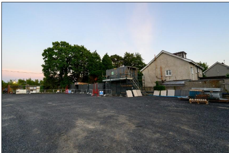
Plate 4 Hardstanding area and construction compound near the site entrance.
