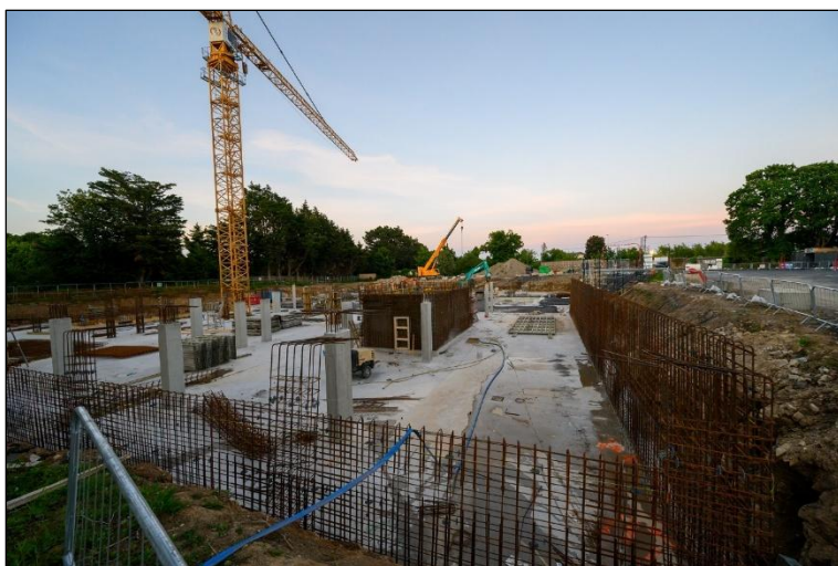
Plate 1 Construction works were already underway at the site at the time of the current survey.
