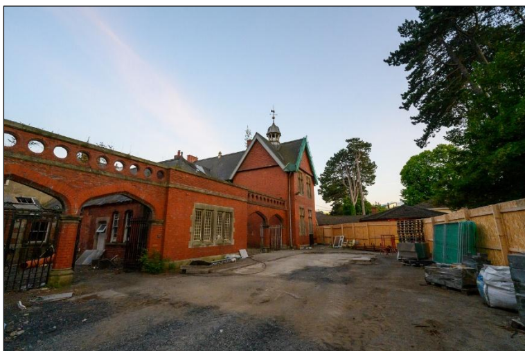
Plate 7 View of the northern side of St. Joseph's house, June 2025.
