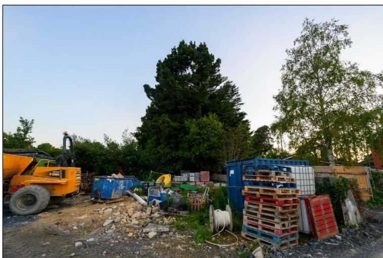
Plate 3 Construction disturbance on the site at the time of the current survey.
