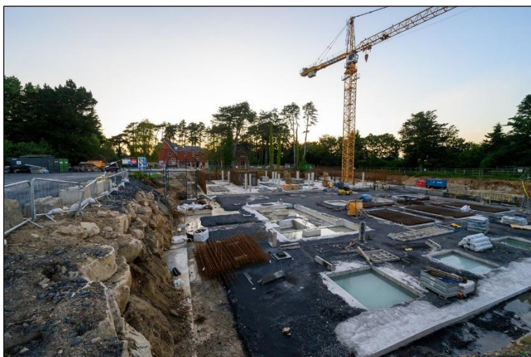
Plate 2 View of the site with St. Joseph's House in the background. Extensive construction works on the site were ongoing at time of the survey.
