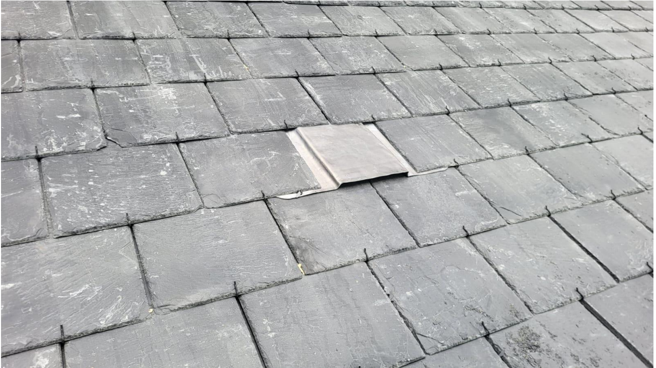
Bat slate in new roof (29.4.2025) of Coole Park Visitor Centre, Gort, Co Galway.
