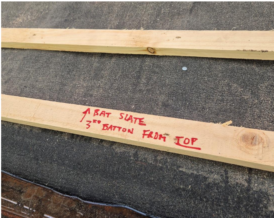
Bat specialist marked up where bat slates (x5) are to be positioned in consultation with NPWS – Coole Park Visitor Centre, Gort Co. Galway.
