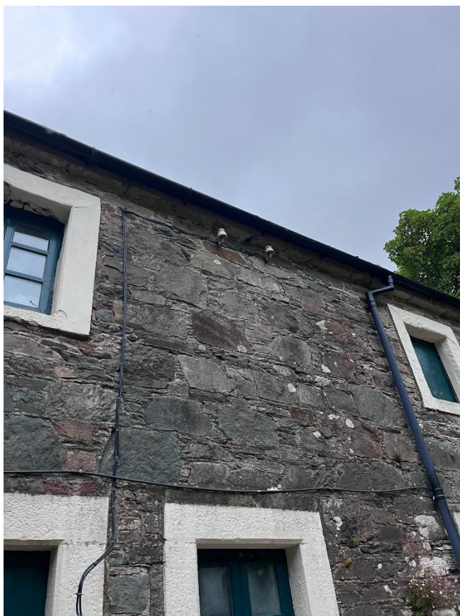
Plate 1 Eastern facing wall at front of building.
