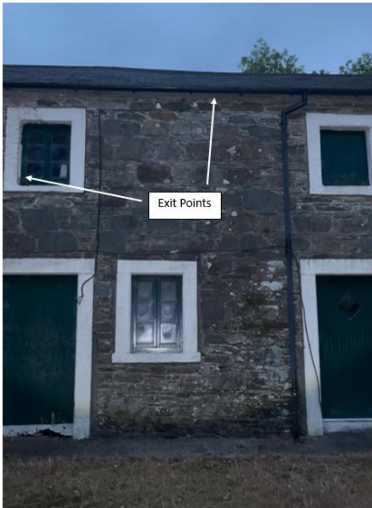
Figure 2 Location of roost/exit points at the front of the building, facing east.
