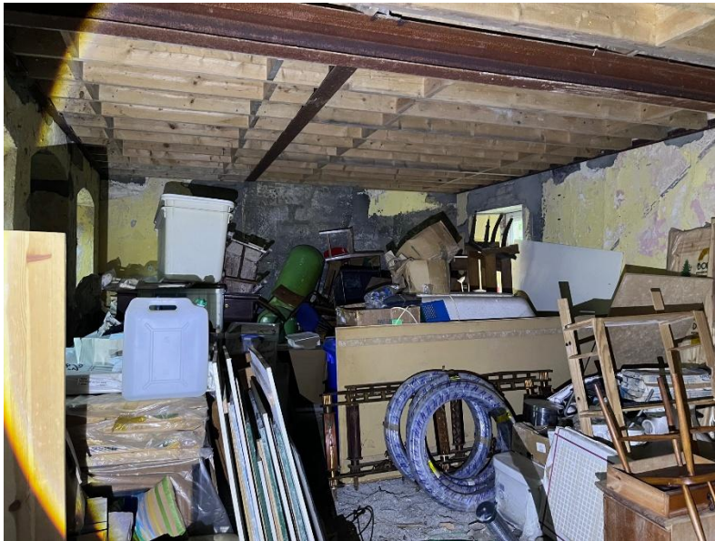
Plate 4 Ground floor of building below the identified roost.
