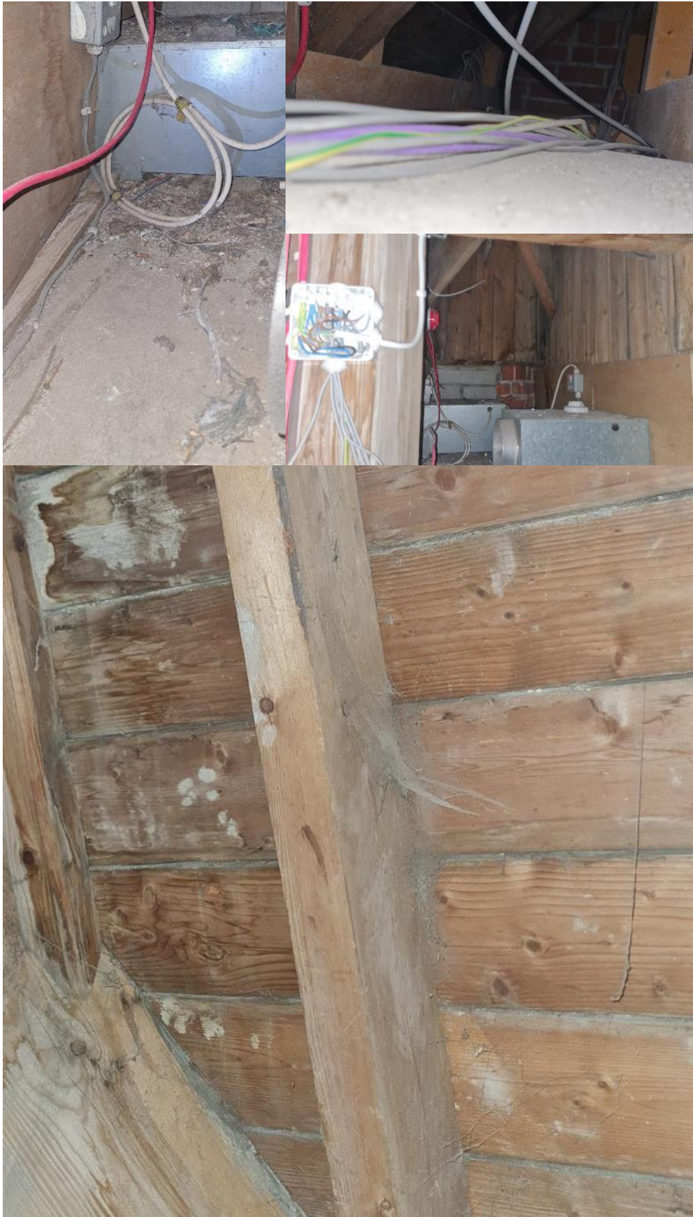
Attic to the south of the proposed lift area. There are no signs of bat usage of this area of roof
