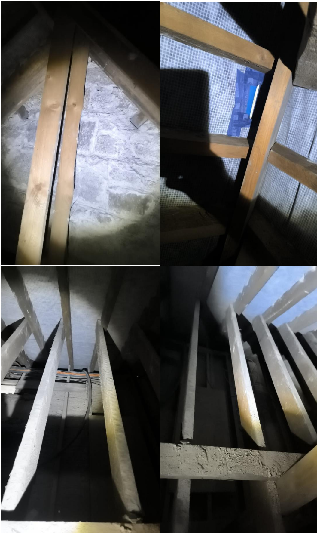
Attic above the proposed lift area
