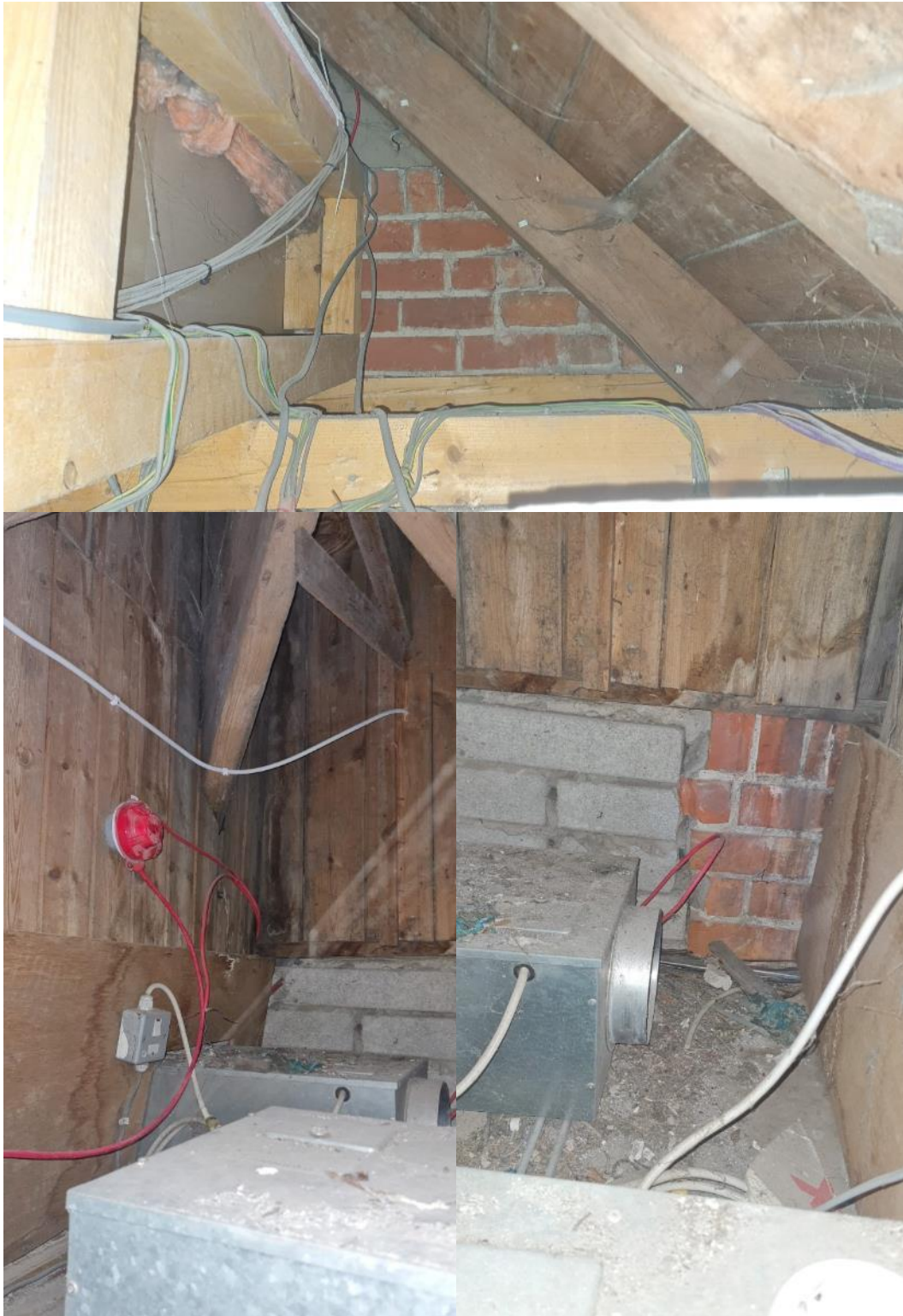
Attic to the south of the proposed lift area. There are no signs of bat usage of this area of roof
