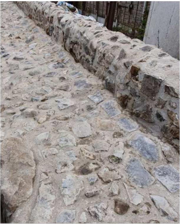
Sample of wall top finish
