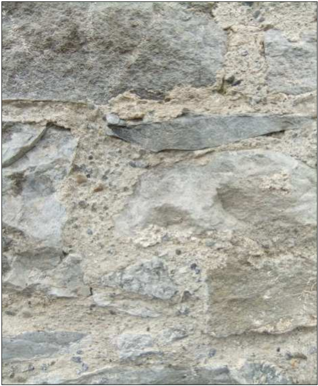
Exemplar provided of flush pointing in stonework beaten back to expose aggregate
