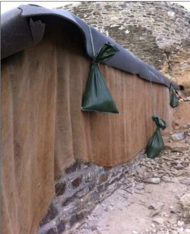
Example of appropriate protection to allow wall to dry out yet not become saturated by rain on upper surfaces
