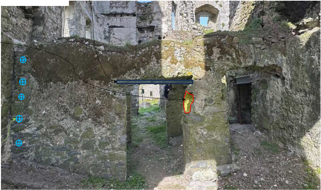
INTERNAL WALL 1 - LOOKING NORTH
