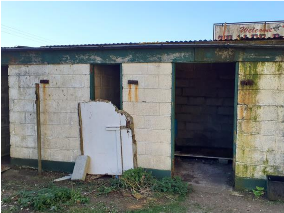
Plate 11. - No.4 - Working Entrance Building
