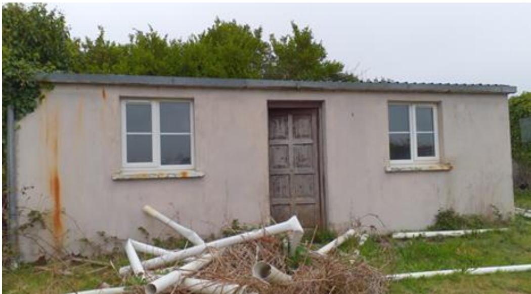
Plate 16. No. 12 - Ancillary building no.4
