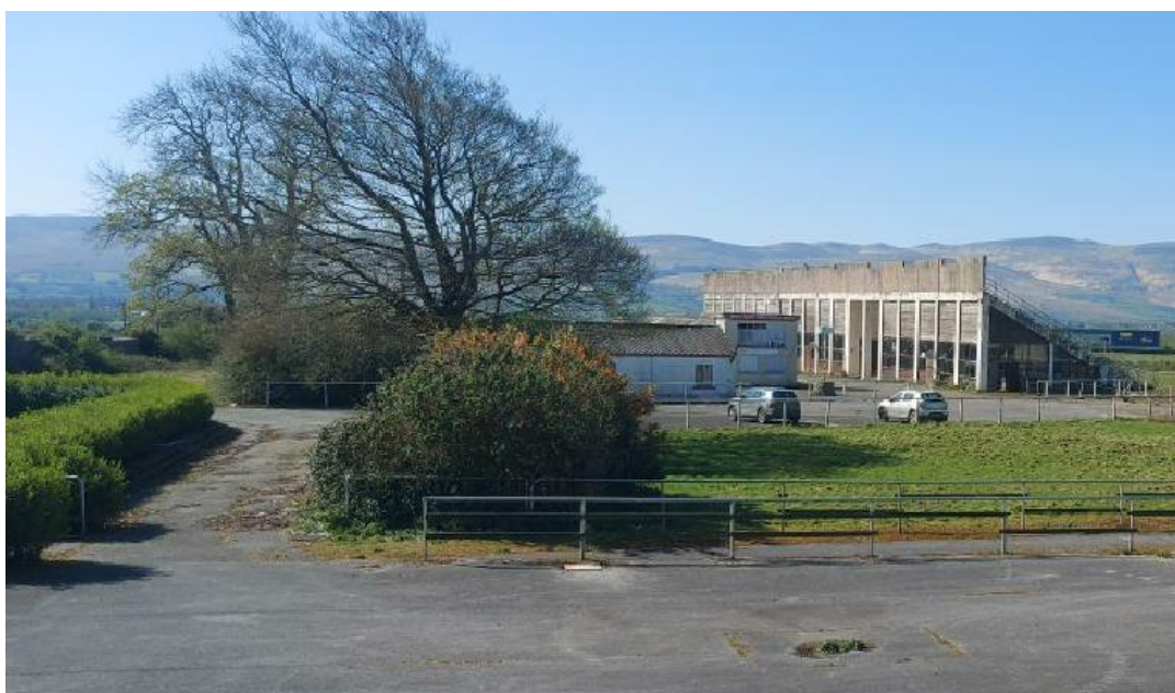
Figure 6. View from Building No. 14 Looking Southwards
