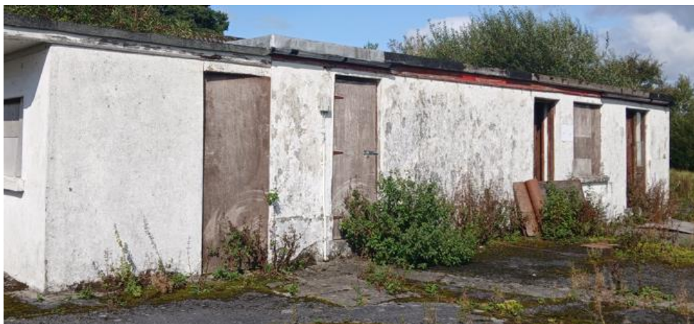
Plate 13. No.9 - Ancillary building no.2
