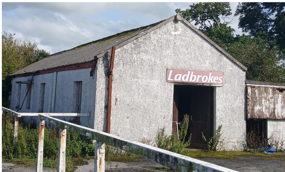
Plate 14. No.10 - Ancillary building no.3
