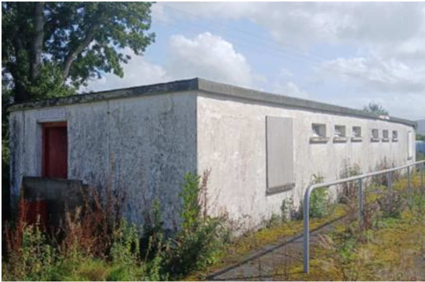
Plate 8. No.3 - Ancillary Building no. 1
