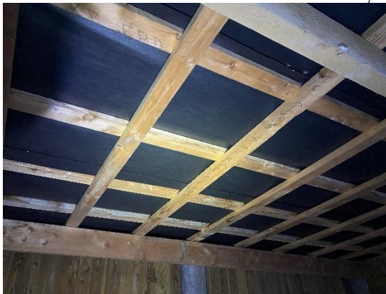
Plate 3-2 Felt lining and timber framing within weather shelter
