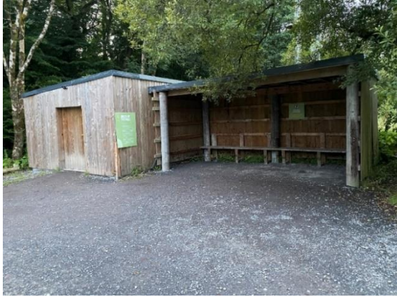
Plate 1: North-eastern aspect of wooden shed and adjoining weather shelter
