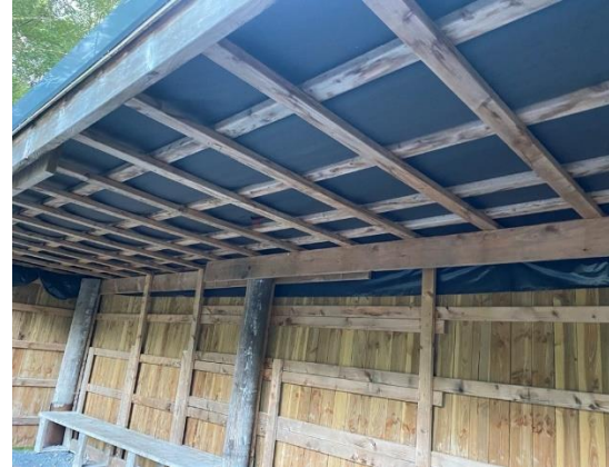
Plate 3-5 Timber framing and felt underlining
