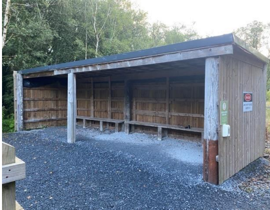
Plate 3-4 North-East aspect of weather shelter
