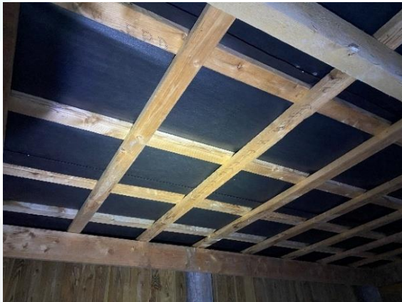
Plate 0 Felt lining and timber framing within weather shelter
