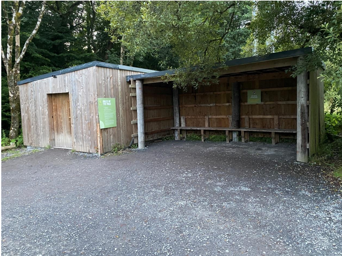
Plate 3-1 Wooden shed and weather shelter north-eastern aspect
