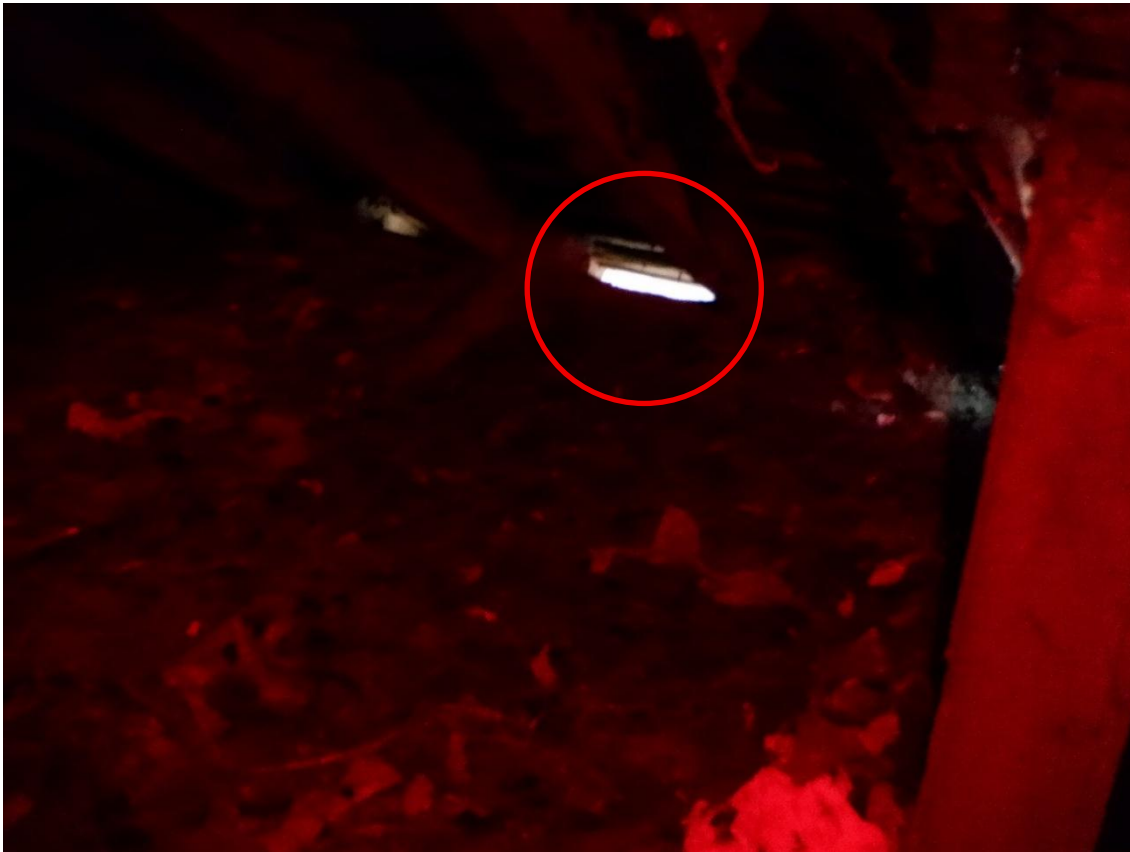
Figure 4-2: Gap under the eaves of the roof providing access to the attic.
