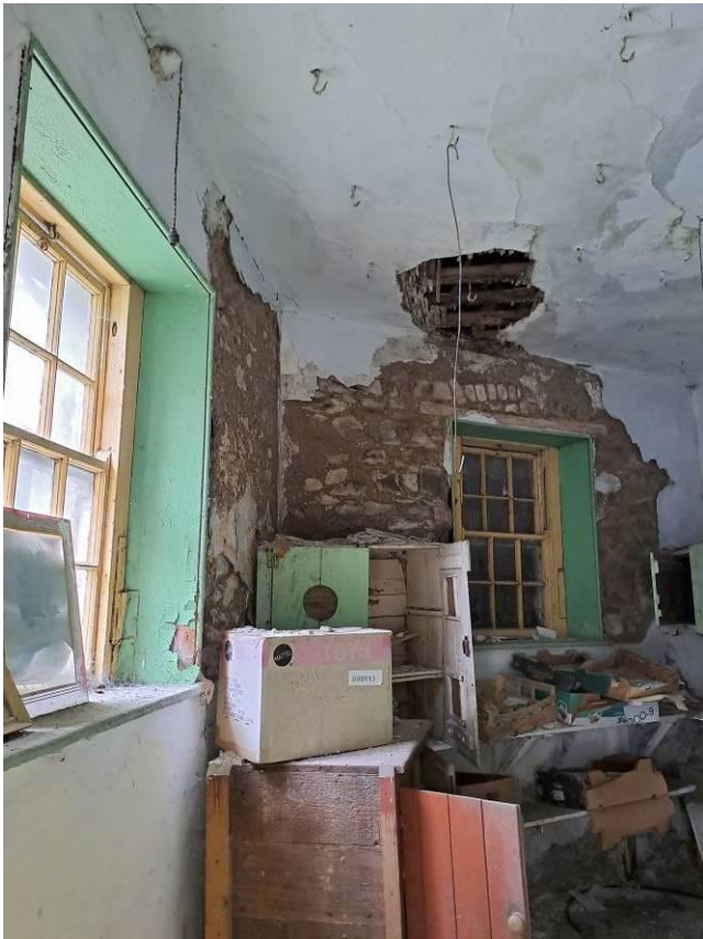
Photo 21: Damp Patch in Ceiling
