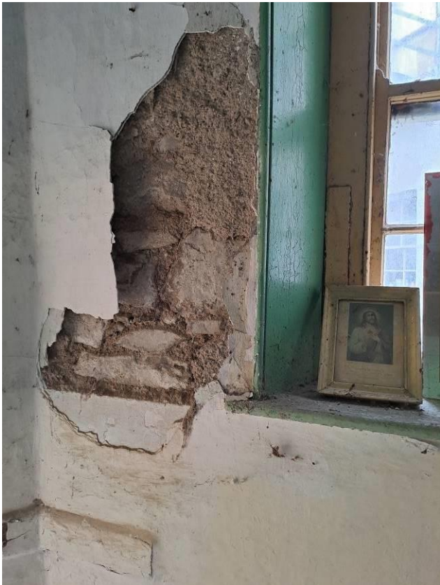
Photo 22: Plaster Cracking
