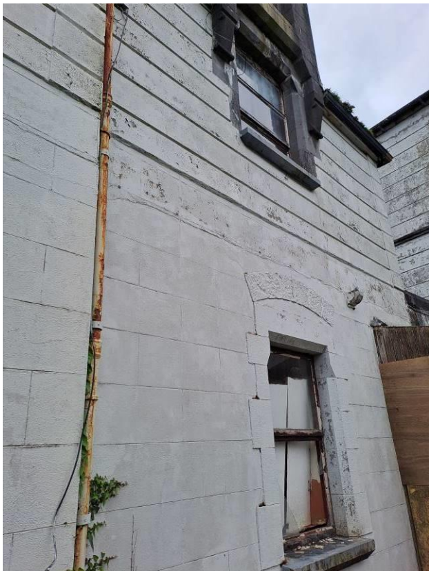
Photo 6: Downpipe Rusting
