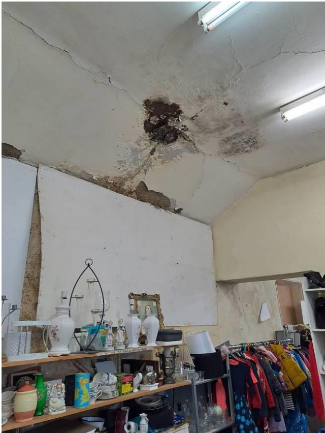
Photo 21: Damp Patch in Ceiling
