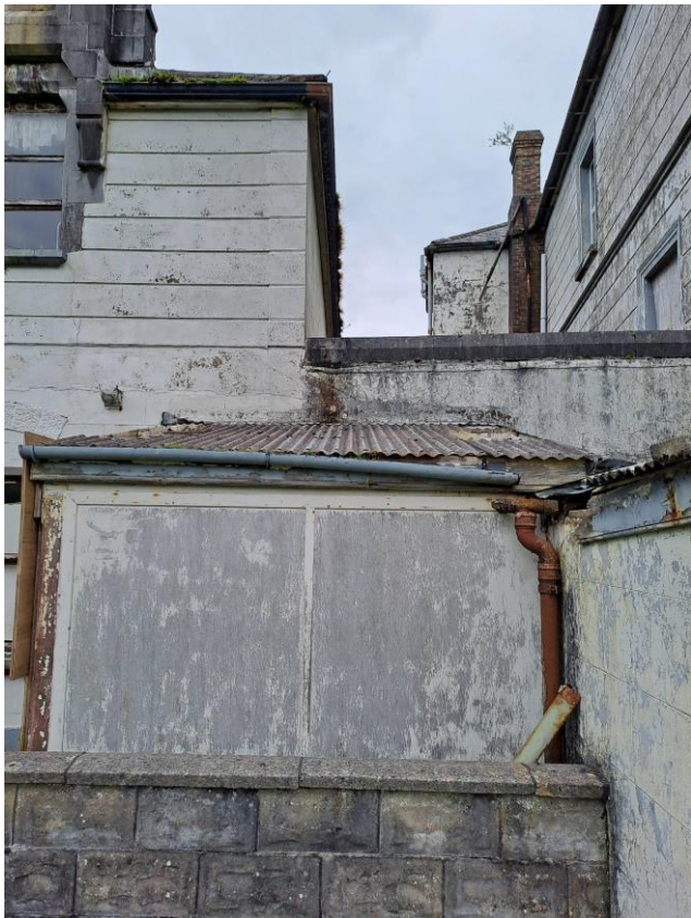
Photo 7: Gutters Blocked
