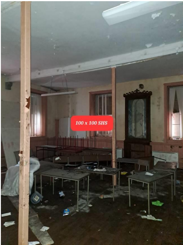
Photo 21: 2 No. 100x100 SHS Sections Supporting Beams Above
