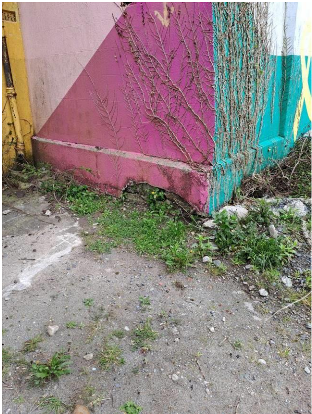
Photo 10: Plaster Broken
