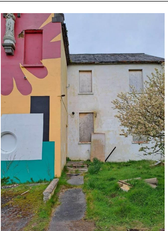
Photo 2: Windows Boarded Up
