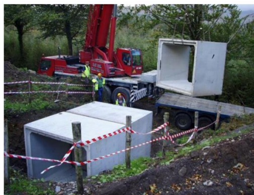
Plate 6.2: View of Flahive Hibernaculum under construction
