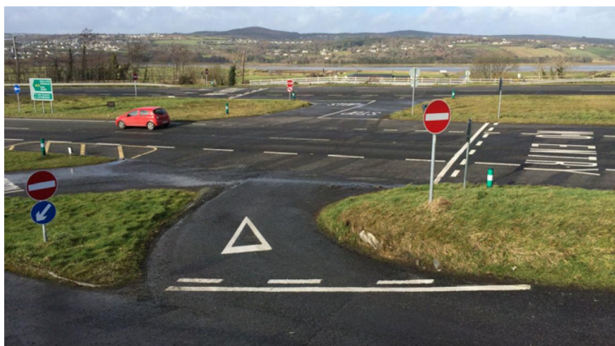
Figure 2.4: Trimragh Junction on the N13 Dual Carriageway
