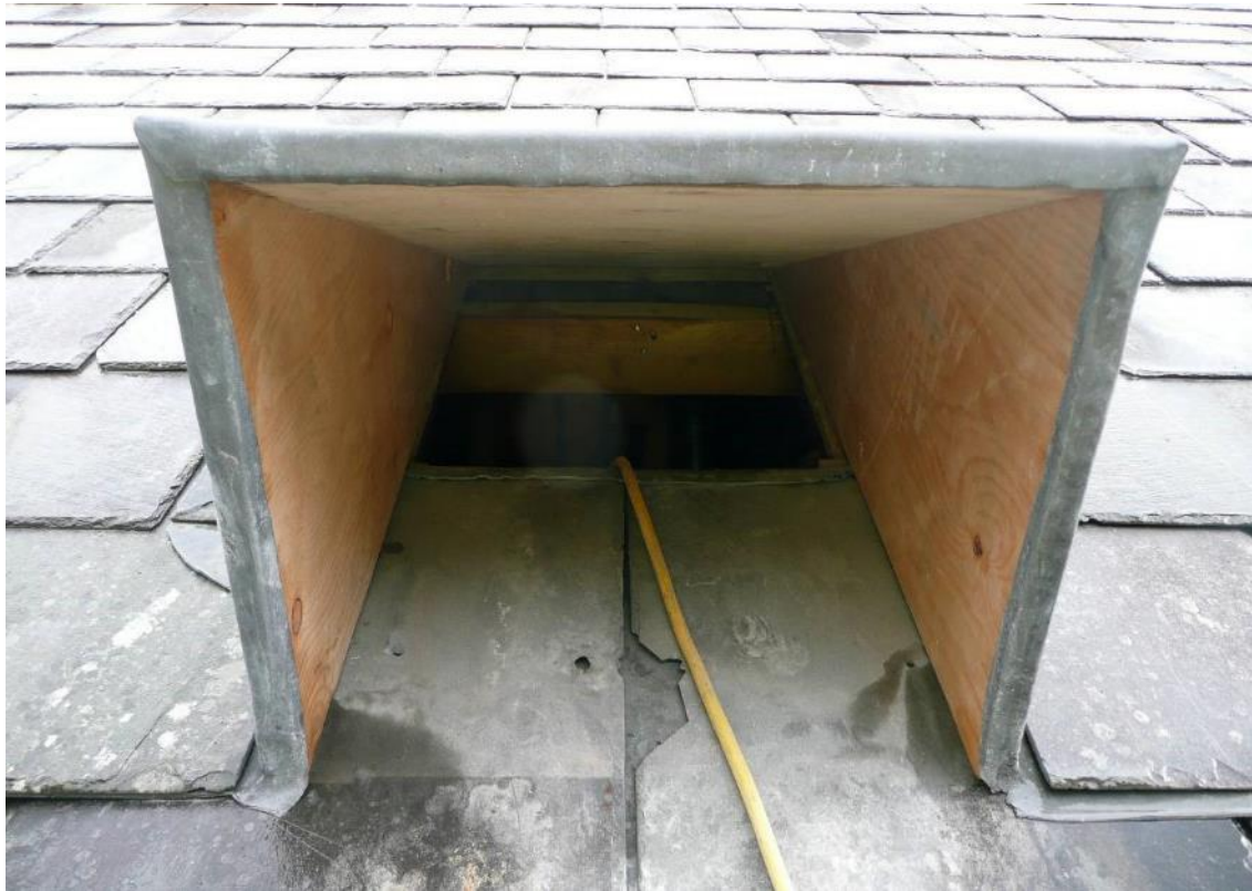
Plate 29: Example of constructed bat roost entrance
