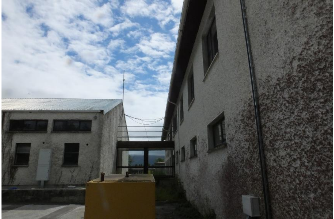
Plate 2: The corridor joining the two office buildings
