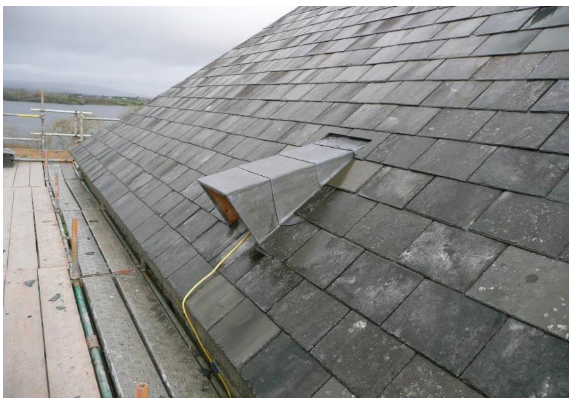
Plate 28: Example of constructed bat roost entrance
