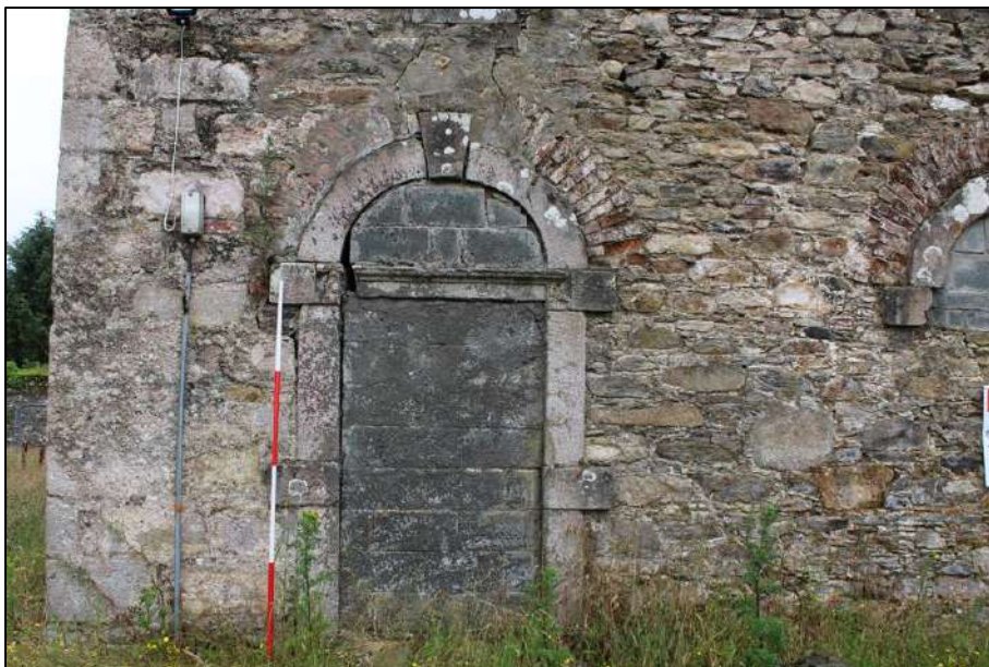
Plate 26: Close up of easterly doorway, note the granite quoins in the eastern gable.
