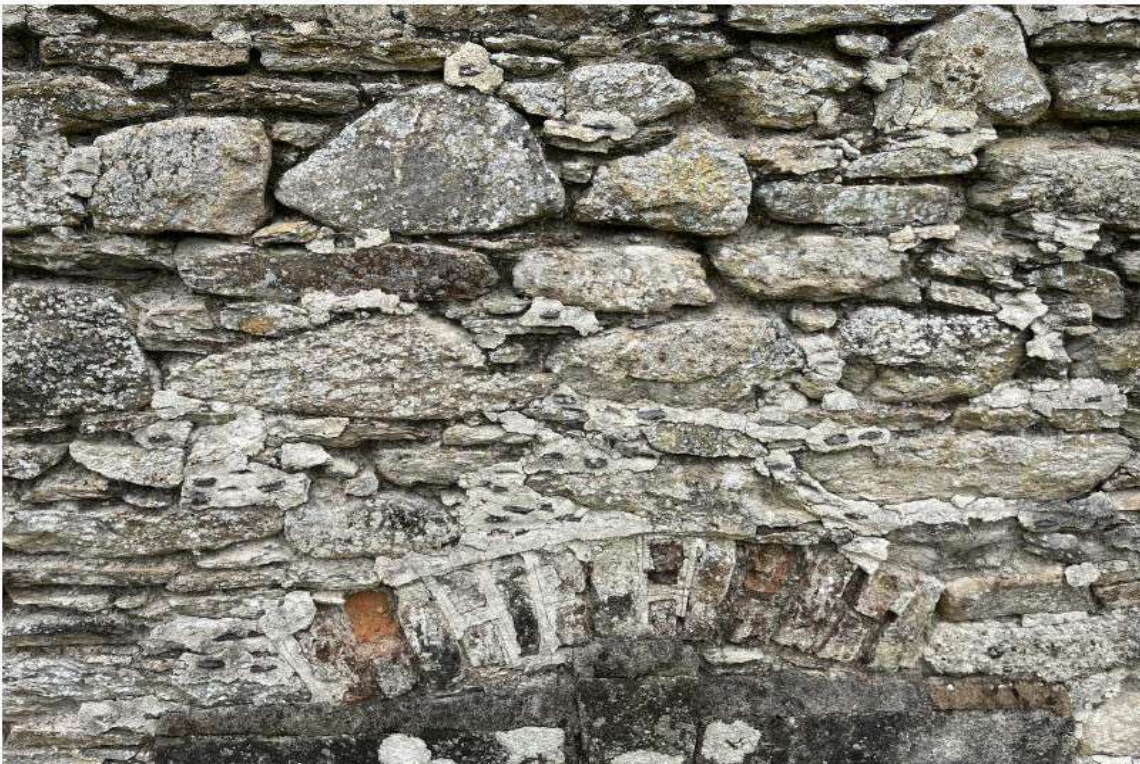
PHOTOGRAPH 4 - FAILED REPOINTING
