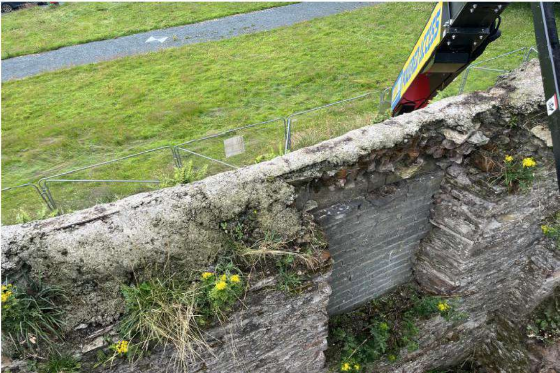
PHOTOGRAPH 6 – CONCRETE FLAUNCHING AT COLLAPSED SECTION OF WALL
