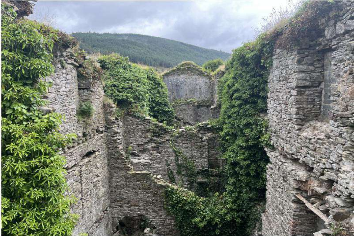
PHOTOGRAPH 17 - COLLAPSED CROSS WALL
