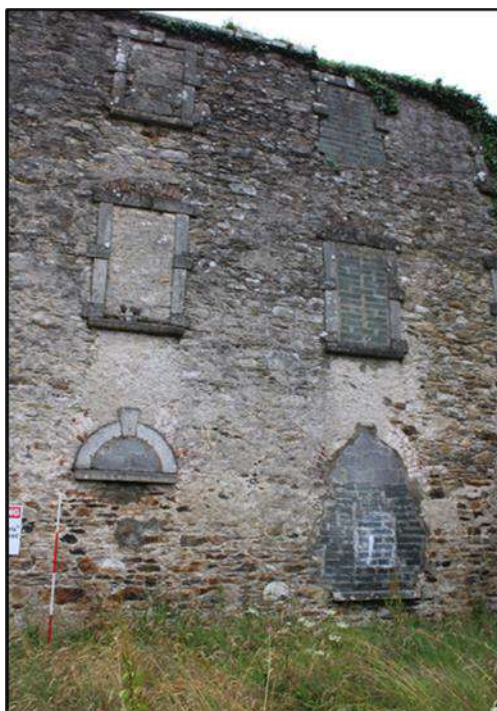
Plate 33: Window which has been enlarged, presumably for access once that barracks was a ruin.
