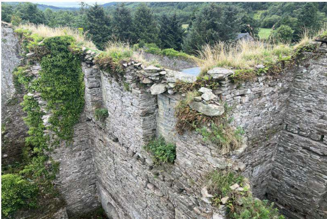
PHOTOGRAPH 12 - SOUTH ELEVATION LOOSE MASONRY AT WALL TOP
