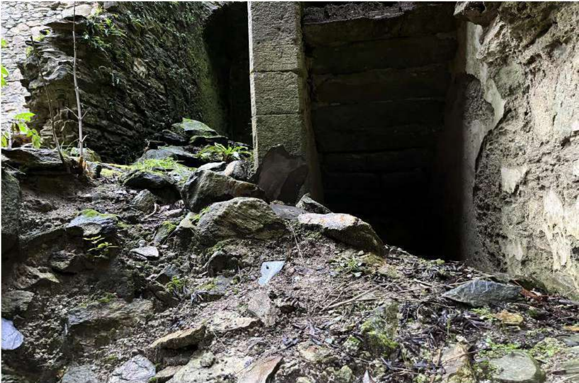
PHOTOGRAPH 19 - COLLAPSED STAIR AT WEST END
