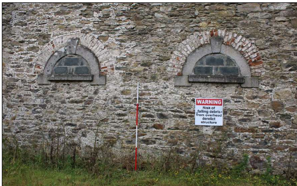
Plate 28: Semi-circular window openings at ground level on north elevation, front of barracks, note the harling with small stones embedded into the mortar.
