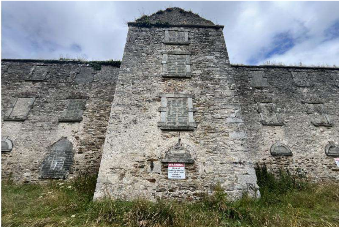
PHOTOGRAPH 11 - SOUTH ELEVATION - STAIRWELL- NOTE SURVIVING HARLING
