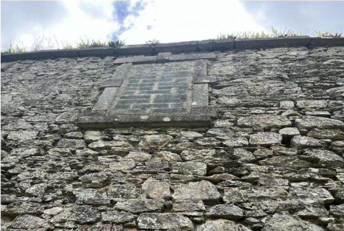
PHOTOGRAPH 3 - ERODED MASONRY JOINTS
