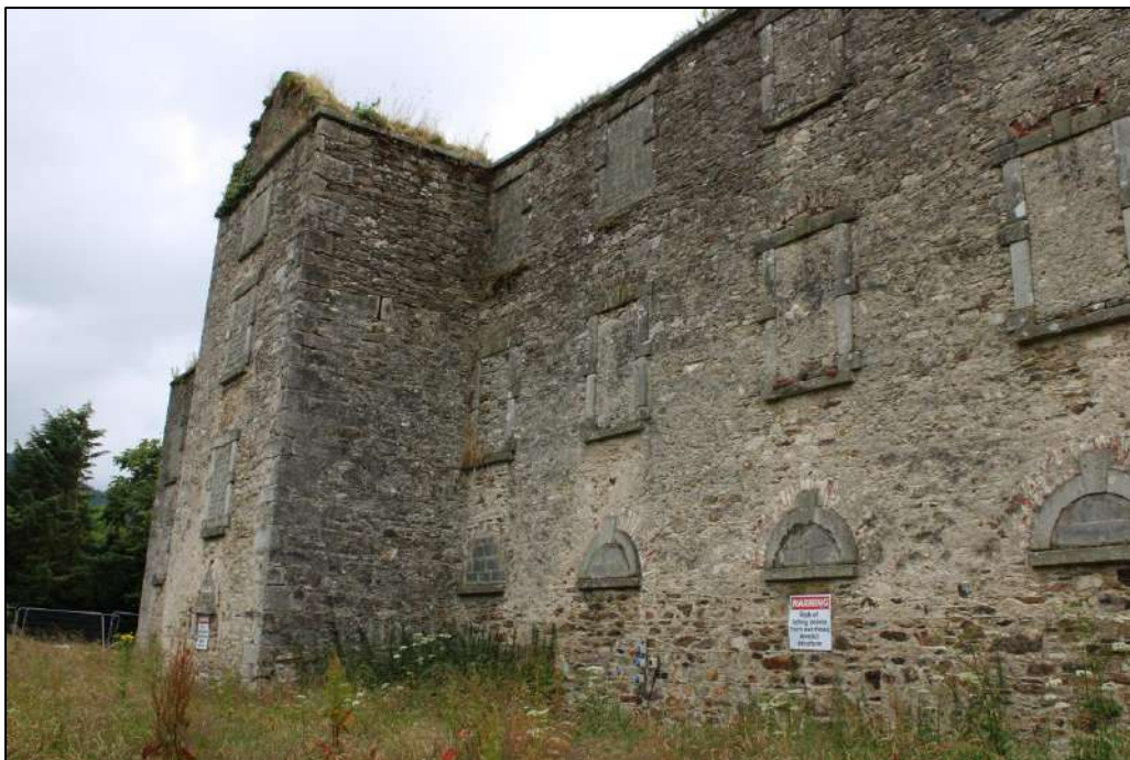
Plate 31: Porch at southern elevation, note the possible gun slit at second floor level.
