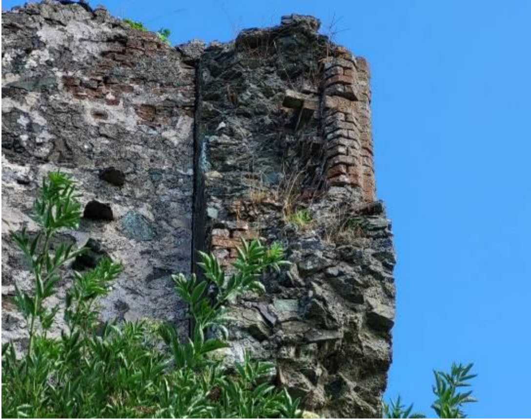
31. South wall exterior – stub of demolished east wall
