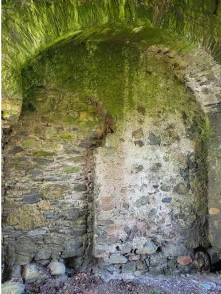
36. Entrance passage – south wall, circular arch at west end (note blocked door)
