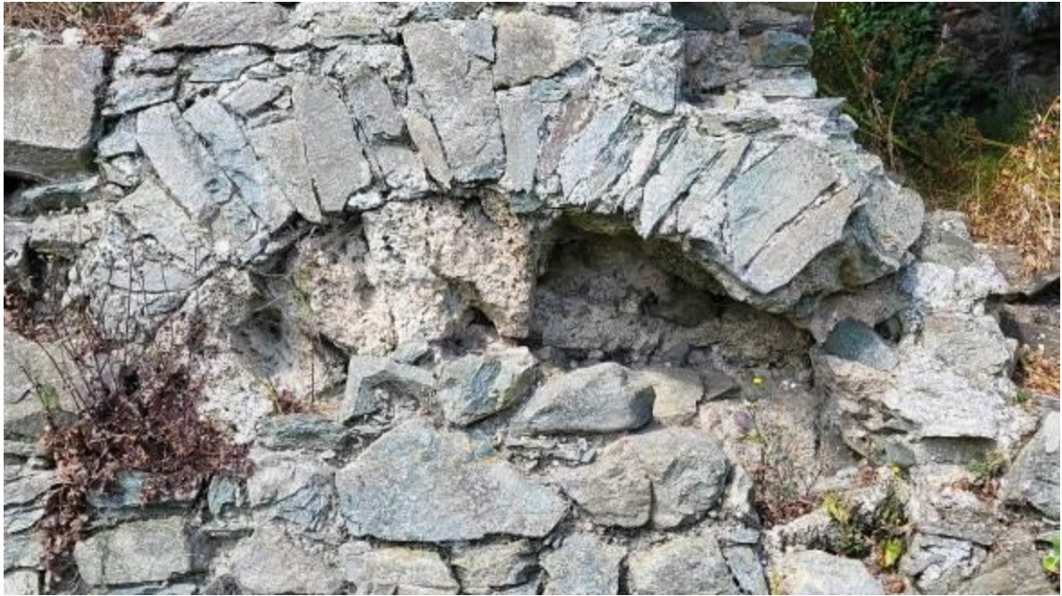
19. East elevation damaged masonry above blocked former entrance – Opening E1
