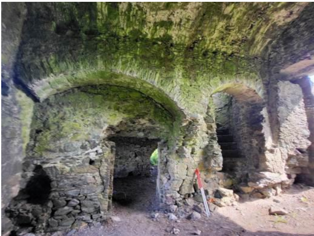
39. Entrance passage north wall – note hole in wall at west end, destroyed pier between arches and degraded masonry at wall base at the east end.
