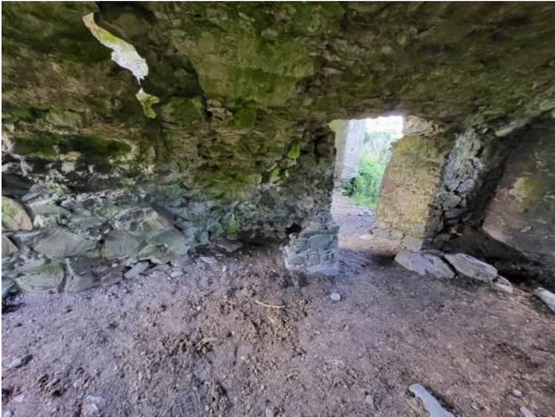
45. Undercroft south wall – note poor arching support to the stairs
