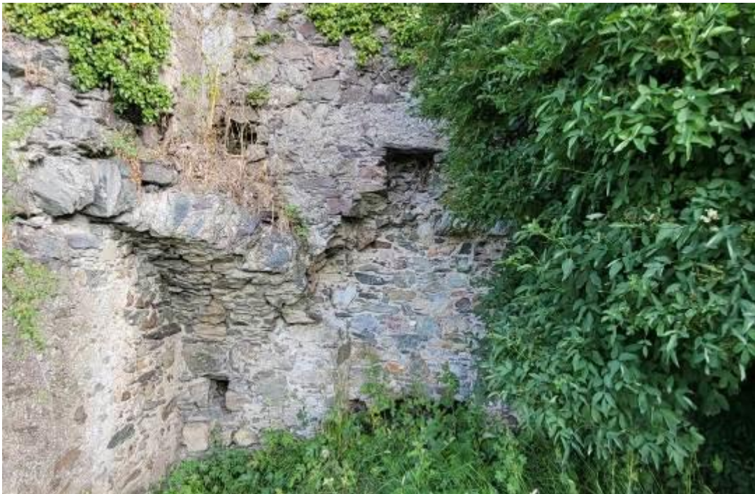
28. South elevation exterior – blocked door Opening S1
