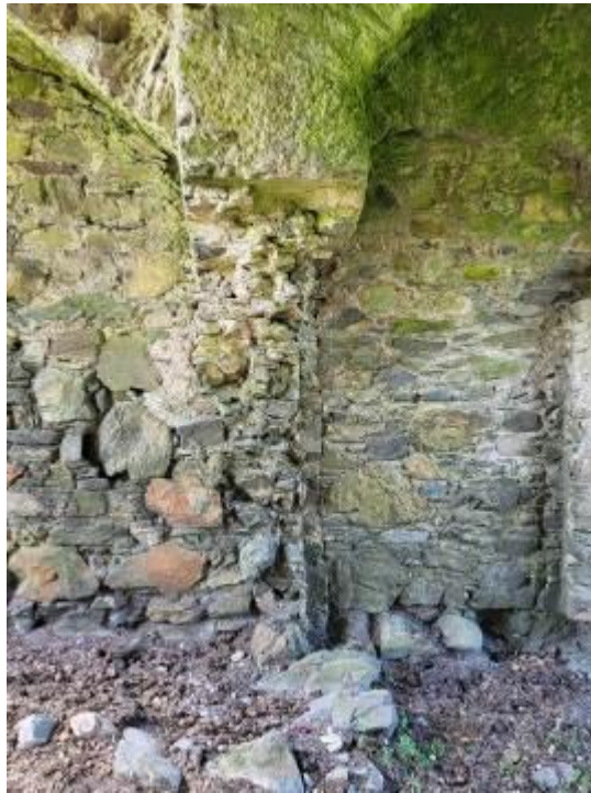
37. Entrance passage – south wall, damaged pier between the two arches
