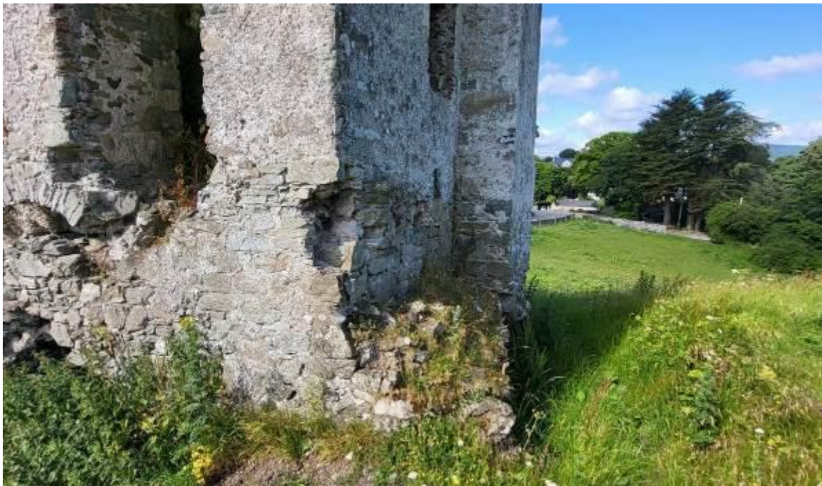
18. East elevation – damaged masonry at north-east corner
