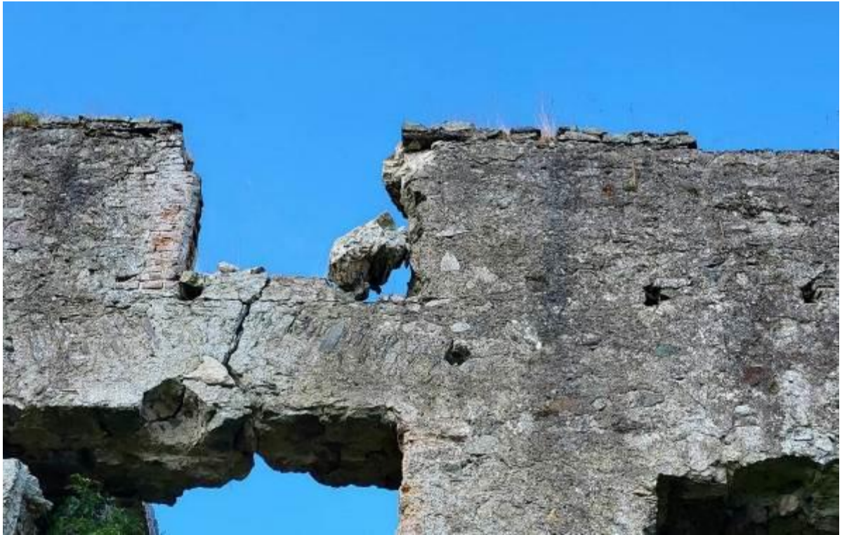
23. East elevation – damaged masonry between Openings E5 and E6
