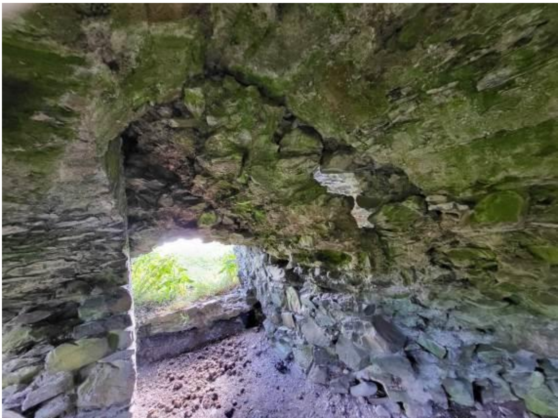
45. Undercroft looking east – note poor arching support to the stairs
