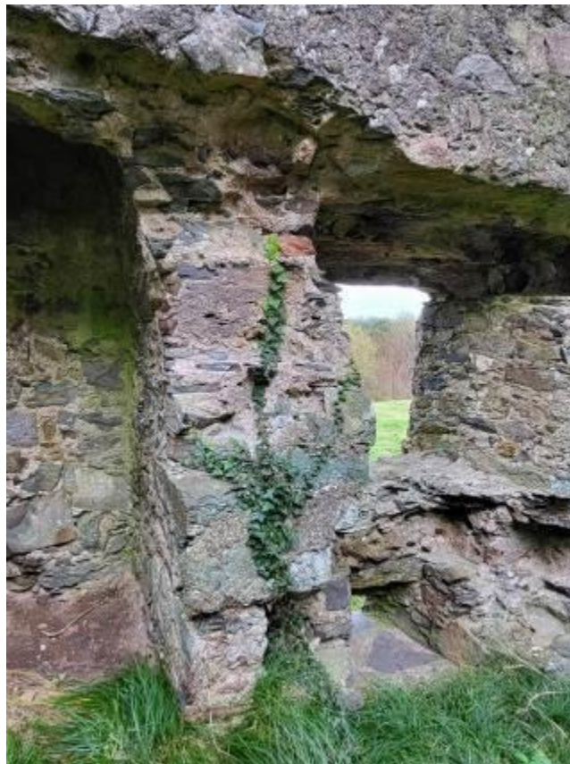
16. North elevation first floor - damaged chimney support wall at window N2
