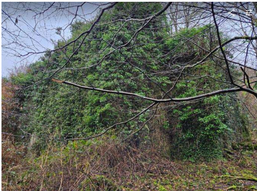
Photo 3- Rear view elevation and side of house facing Templehoe.
