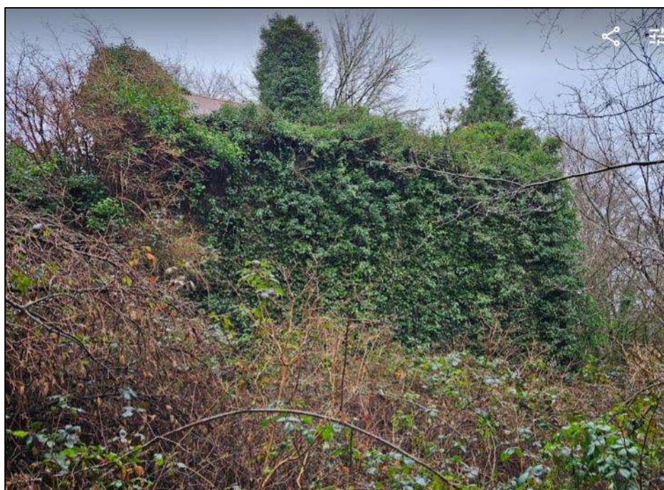
Photo 2: Furze Point House, rear view
