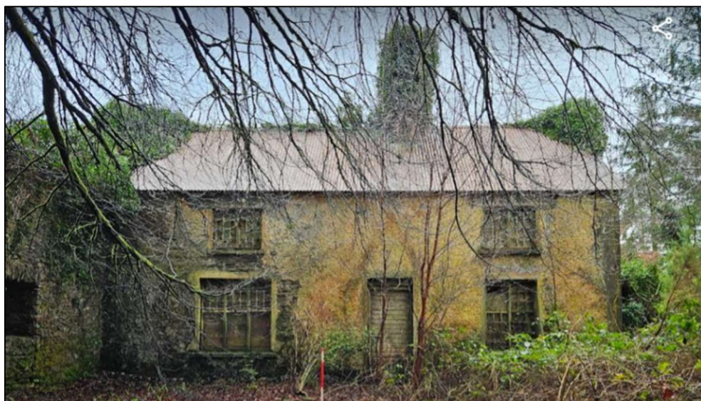
Photo 1: Furze Point House, front view
