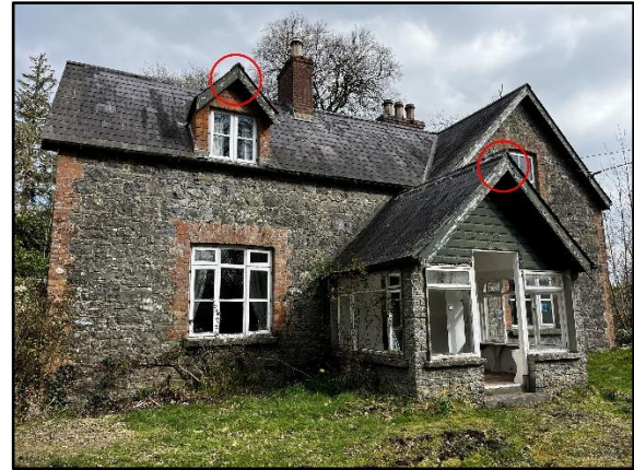
Plate 2: 1no. Soprano pipistrelle emerged from soffit of south facing dormer window (left circle). 3 no. soprano pipistrelles emerged from fascia at apex of porch gable (right circle).
