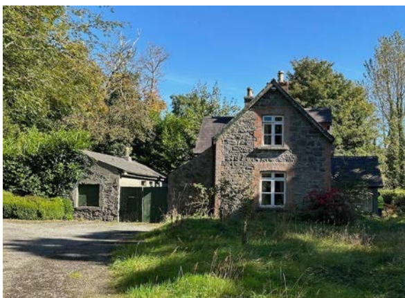
VIEW FROM APPROACH (WEST SIDE)
