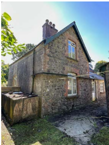
REAR GABLE W/ WATER TANK
