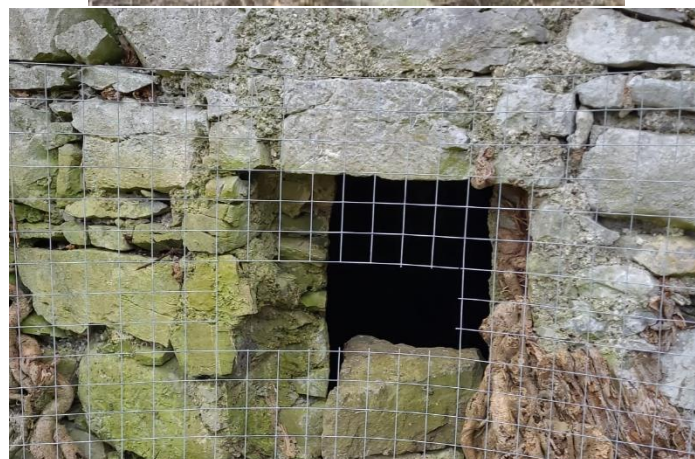
Bat in crevices and retention of bat access
