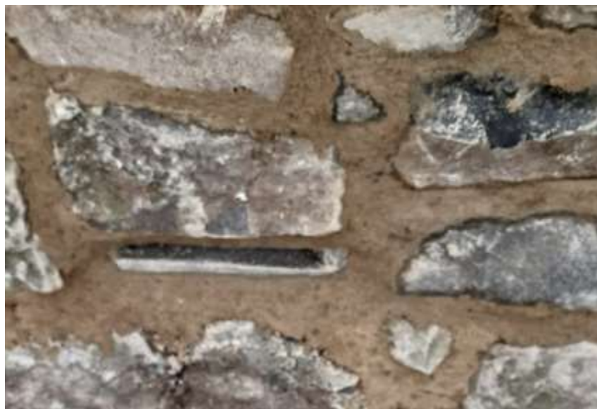
Installed bat tubes.
