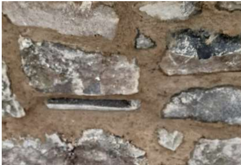
Installed bat tubes.
