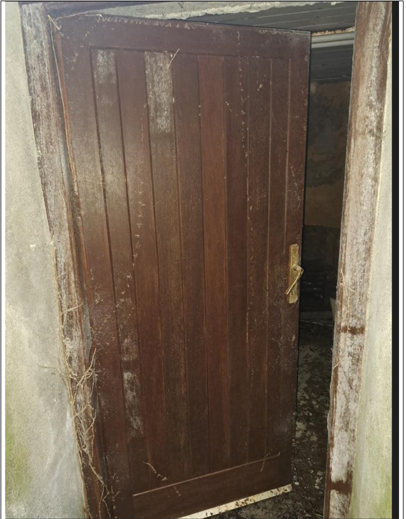
Sand and seal existing timber door to rear of building. Replace all ironmongery including new lock.
