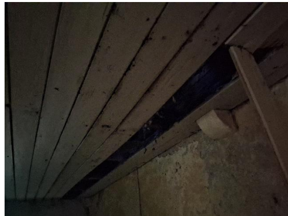
Plate 10 Broken ceiling panel allowing limited visual access into the attic space, as well as a potential access point for bats.
