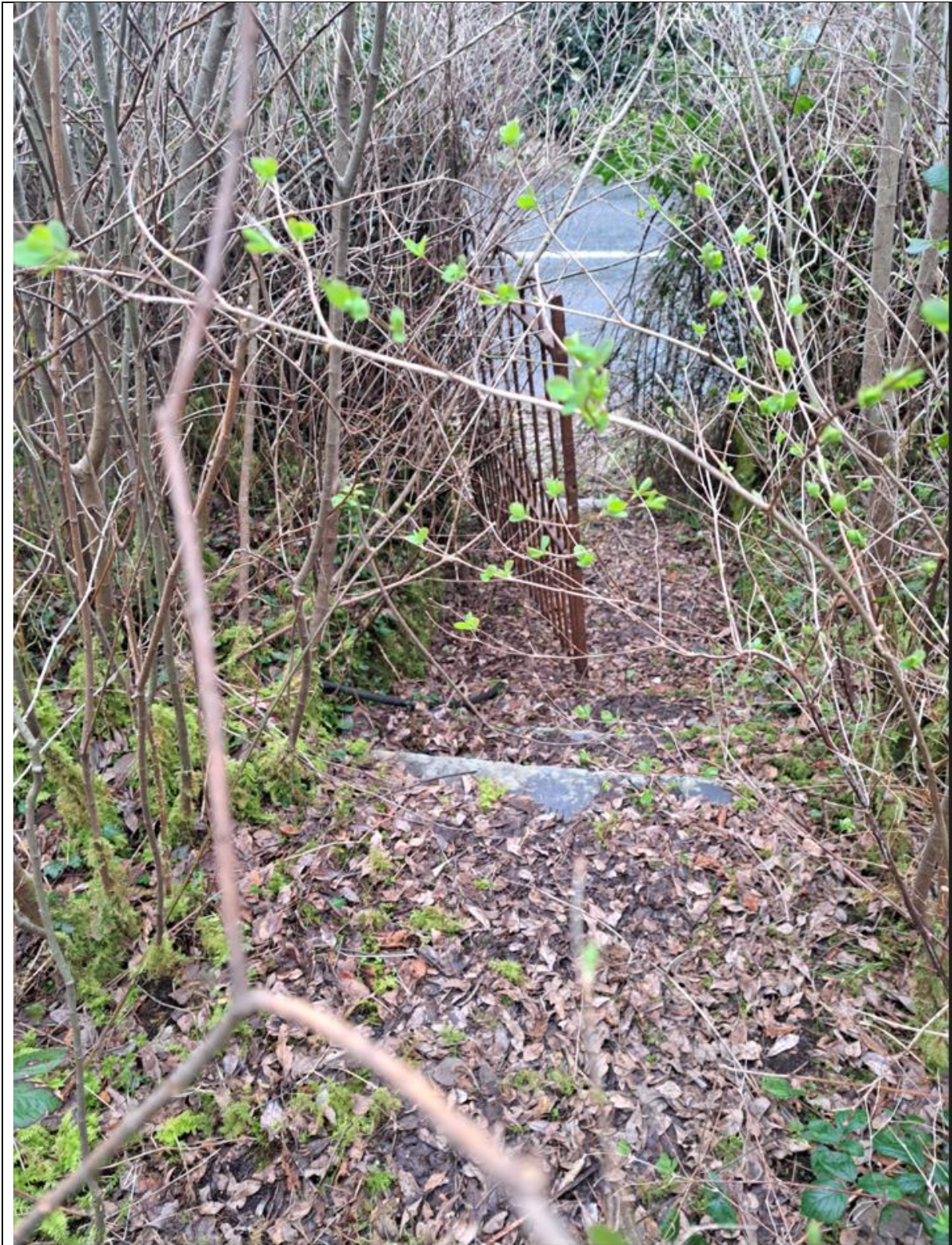
View of the only entrance to the Courthouse property. Clear all vegetation from path and power was area. Relocate 1/2" water mains supply to building so not to cause trip hazard.
