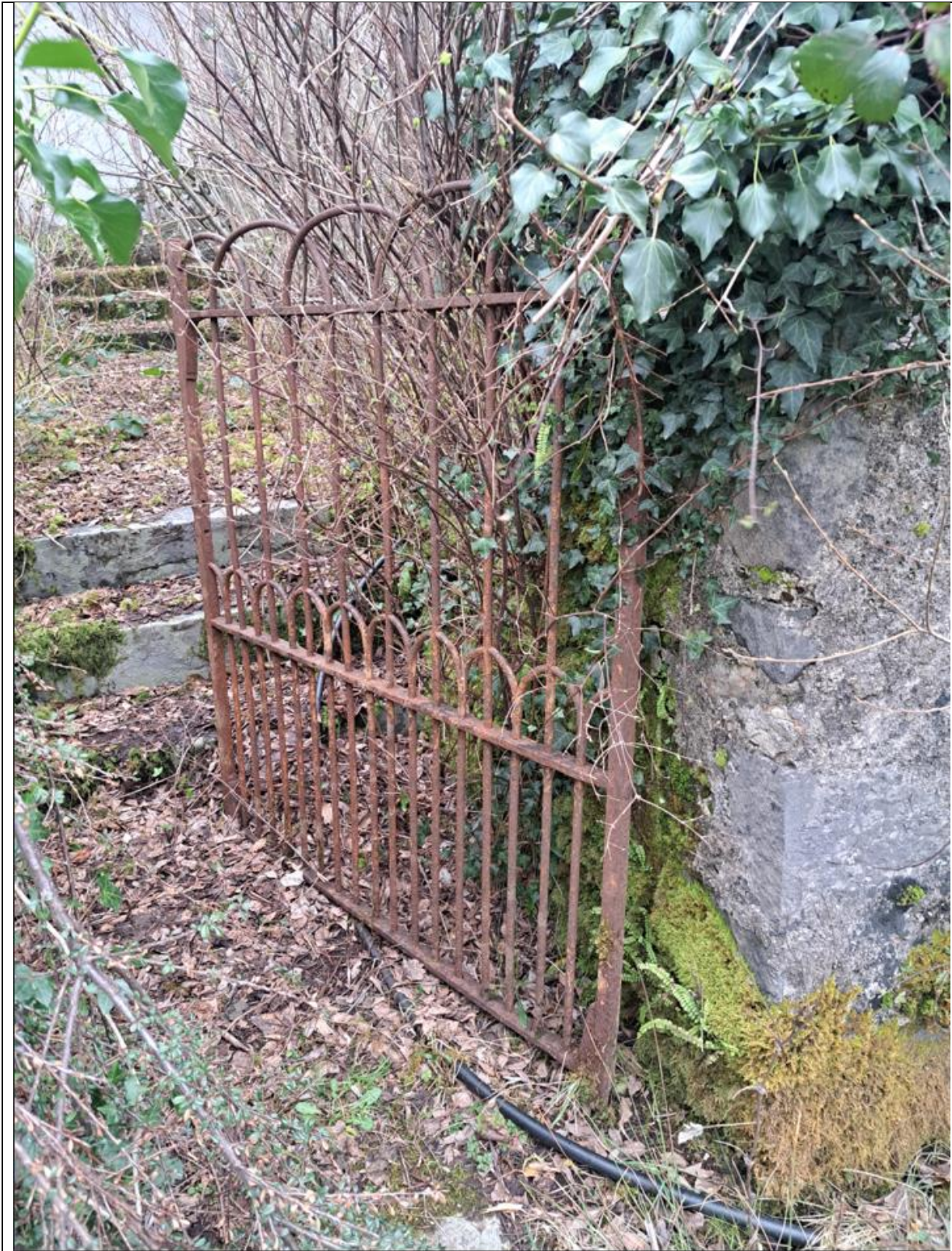
Entrance point to the property. Entrance gate to be removed, treated and re hinged. Ensure gate can only open inwards and not onto the public road. Provide for padlock with access code.
