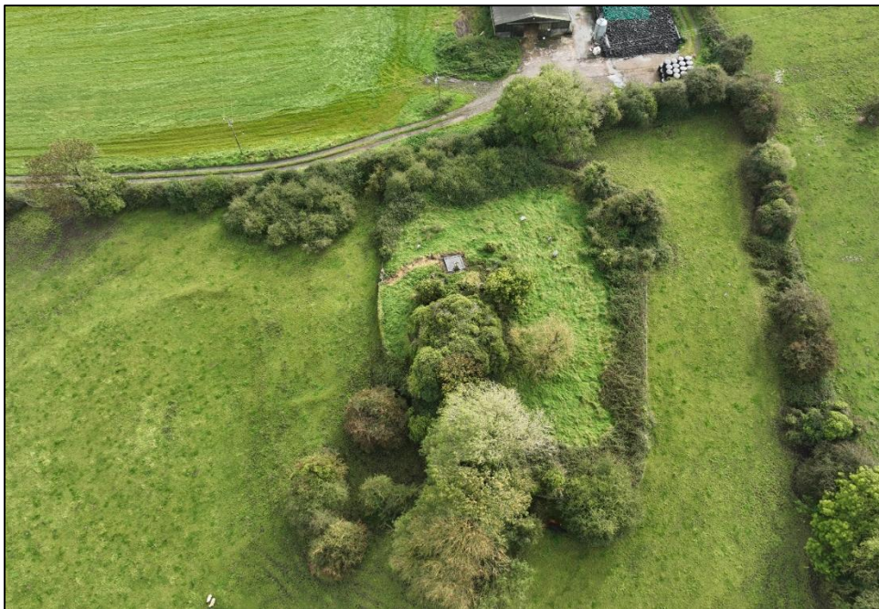
Figure 6: Aerial overview of exterior of structure
