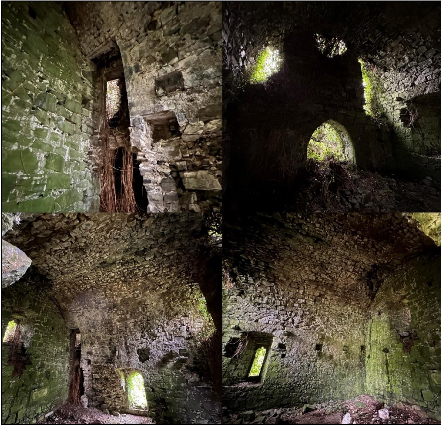
Figure 6: Interior of structure
