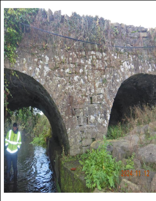
Anti-scour skirting to main arch abutment
