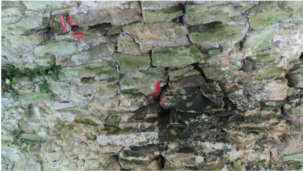
Photo 11 – two additional crevices marked for retention under river arch
