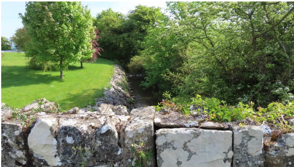
Photo 14 – watercourse upstream lined with rock armour
