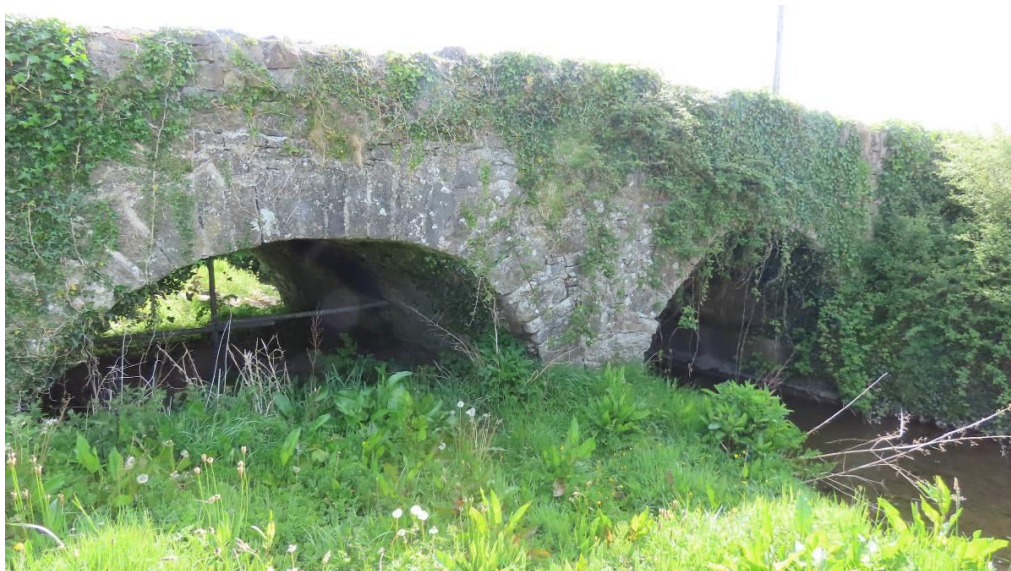
Photo 2 – downstream face of bridge showing dry arch and river arch
