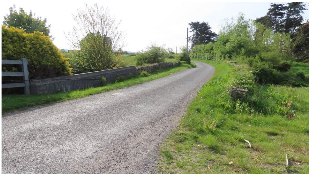
Photo 1 – looking across Ballynoe Bridge
