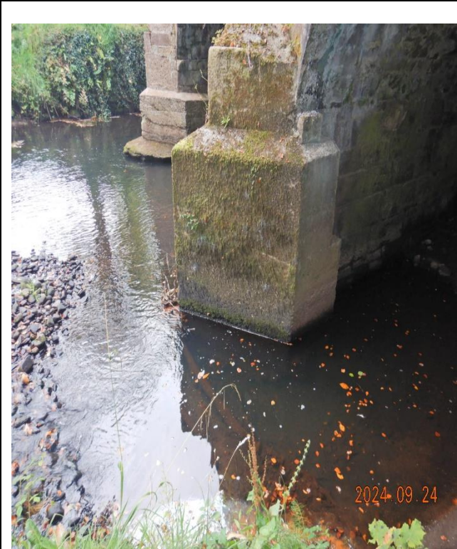
Existing concrete protection to cutwaters
