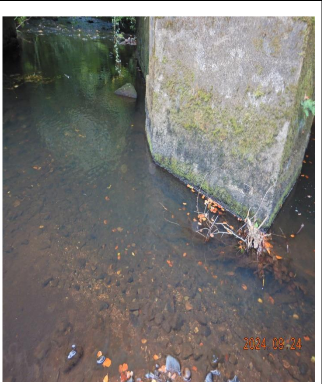
Deep Hole in front of Cutwater – Turbulent Flow
