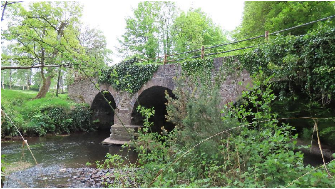
Photo 3 – upstream elevation of Ashroe Bridge
