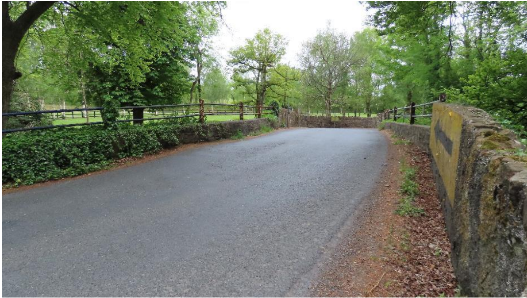
Photo 1 – view over Ashroe Bridge looking south
