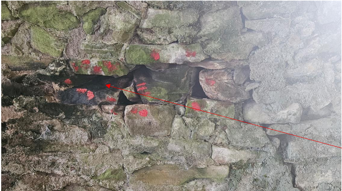
Photo 5 – close up of void used by maternity roost under southern arch
