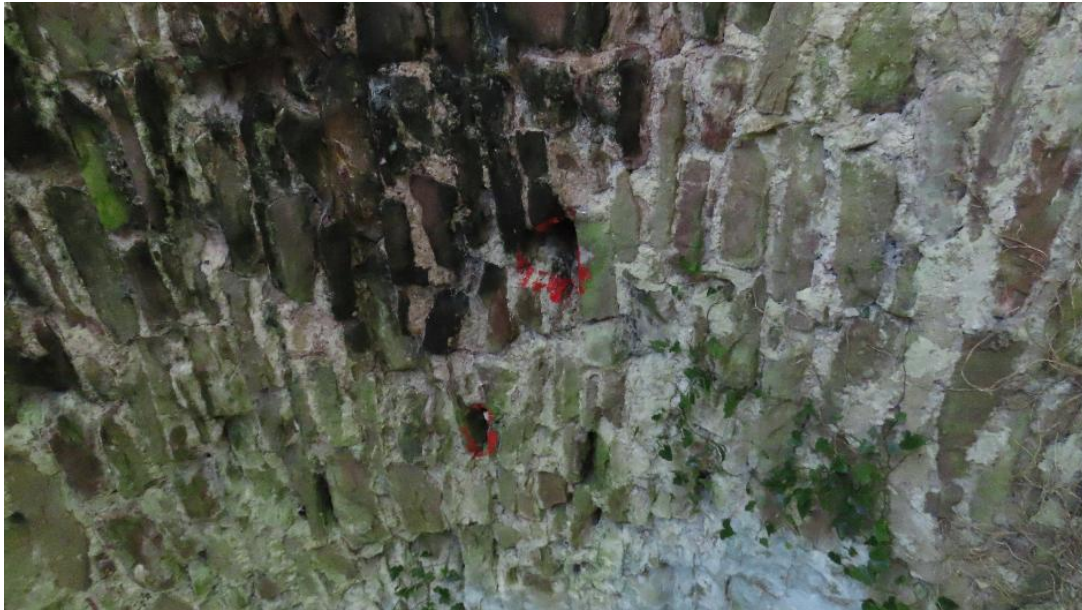
Photo 7 – crevices marked for retention under Arch 3
