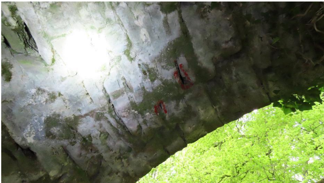
Photo 8 – crevices marked for retention under Arch 3
