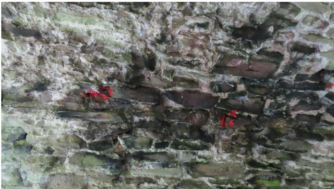
Photo 6 – crevices marked for retention for bats under southern arch (Arch 1)
