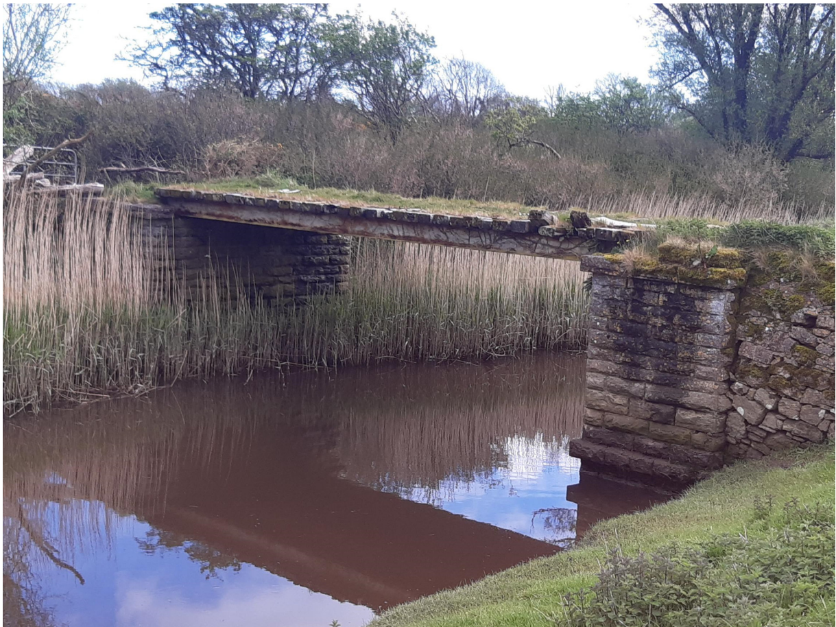
Photo 1 – Bridge structure to be surveyed
