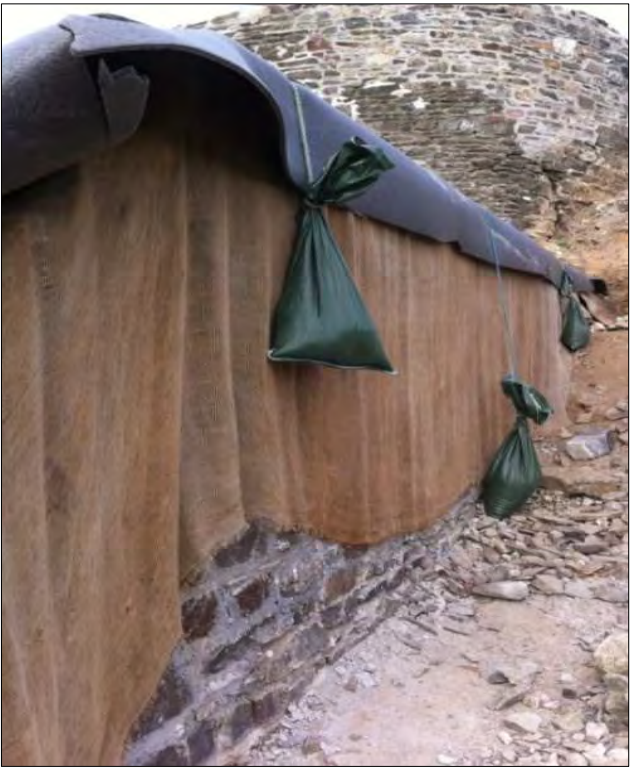
Example of appropriate protection to allow wall to dry out yet not become saturated by rain on upper
