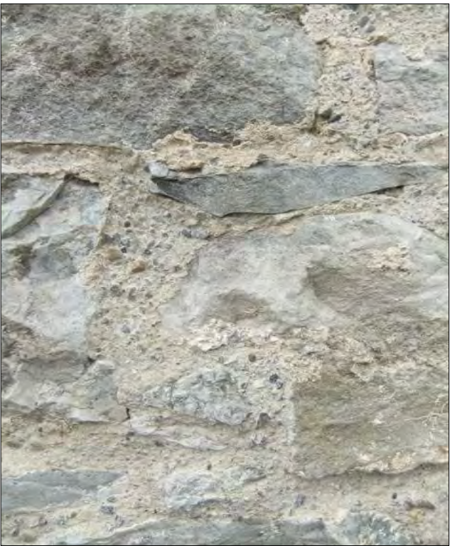
Example of flush pointing in stonework beaten back to expose aggregate
