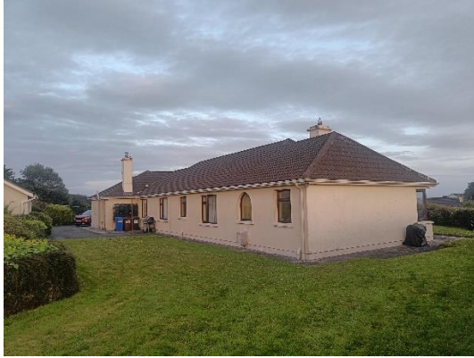
Plate 3-7 Occupied Dwelling, northern aspect.
