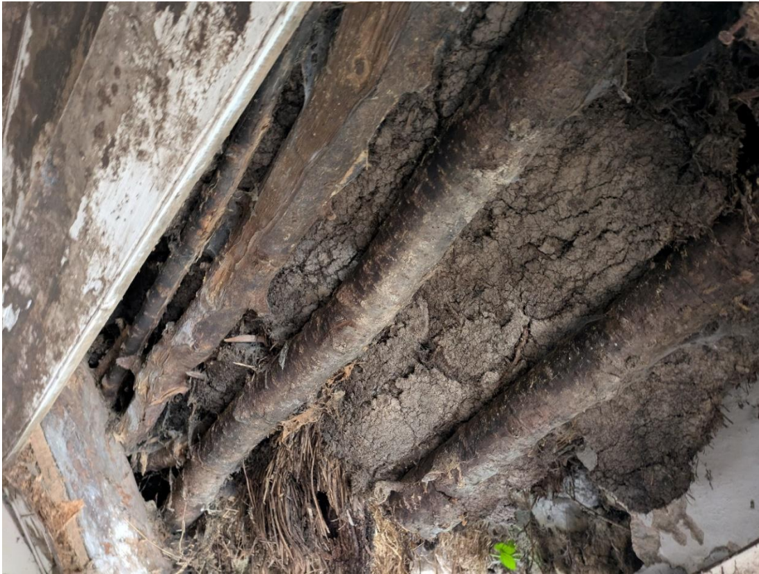
Figure 4-3: Thatched roof visible through collapsing ceiling and wall.
