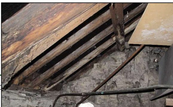
Plate 3. Building A. Ground floor ceiling with rotten timbers and collapsed plaster
