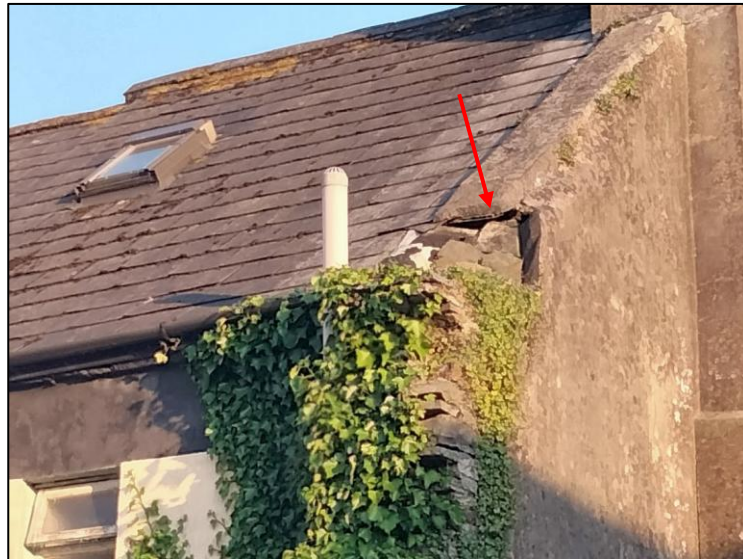
Plate 10. Building B. Rear view of building parapet with hole (red arrow)
