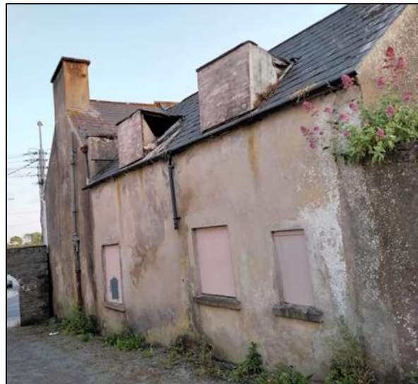
Plate 2. Building A, side elevation with extension (right of photo). Dormers set into roof allow bats easy entry but internal conditions are damp and draughty
