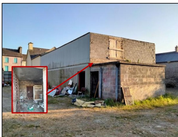
Plate 15. Building C. East facing wall of extension with pitched roof. Building D on right, note holes in stonework and exposed end rafters. Bat roost potential considered medium
