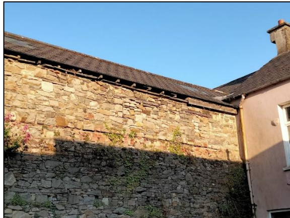
Plate 15. Building C. East facing wall of extension with pitched roof. Building D on right, note holes in stonework and exposed end rafters. Bat roost potential considered medium
