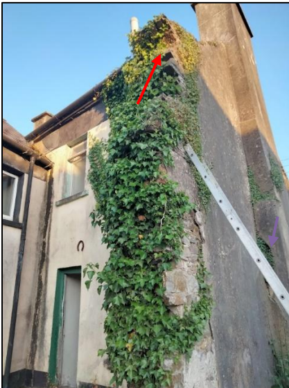
Plate 9. Building B. Rear view of building, parapet with hole (red arrow) and cracks in the wall render (yellow arrow)
