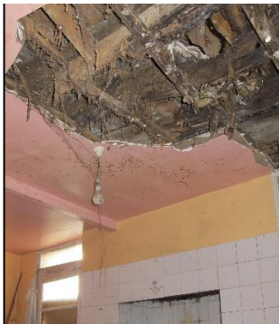
Plate 3. Building A. Ground floor ceiling with rotten timbers and collapsed plaster
