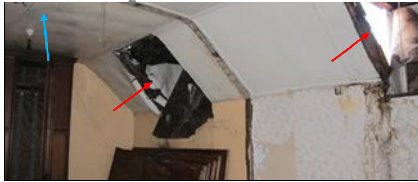
Plate 4. Building A. Internal view of dormers (red arrows). Attic (blue arrow) was not accessible and is limited in height to approx. 1 metre
