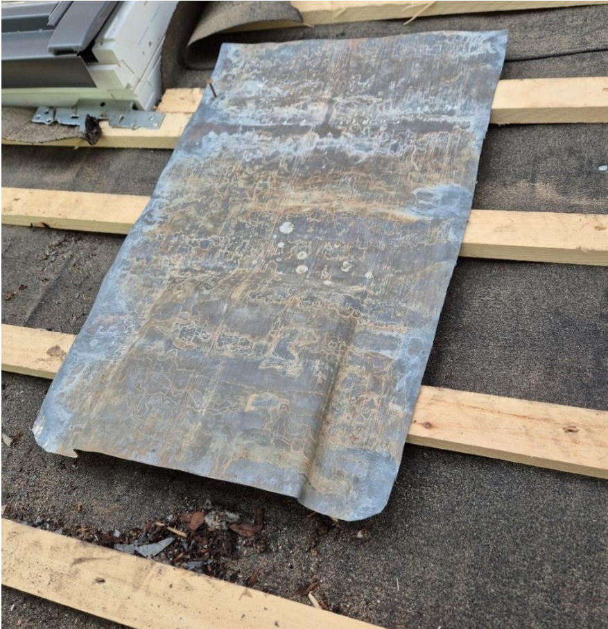
Plate 2a: Construction of bat slates for inspection by bat specialist at Coole Park Visitor Centre, Gort, Co. Galway.
