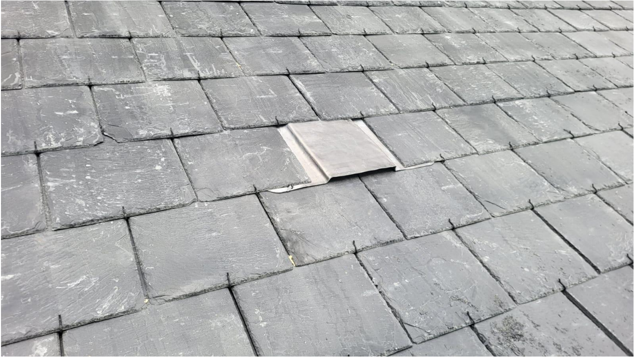
Plate 2c: Bat slate in new roof (29.4.2025) of Coole Park Visitor Centre, Gort, Co Galway.
