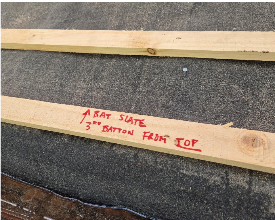
Plate 2b: bat specialist marked up where bat slates (x5) are to be positioned in consultation with NPWS – Coole Park Visitor Centre, Gort Co. Galway.
