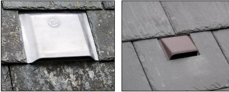
FIGURE 9. EXAMPLE BAT ACCESS TILES / VENTS (JUST LEAD, BEDDOES).
